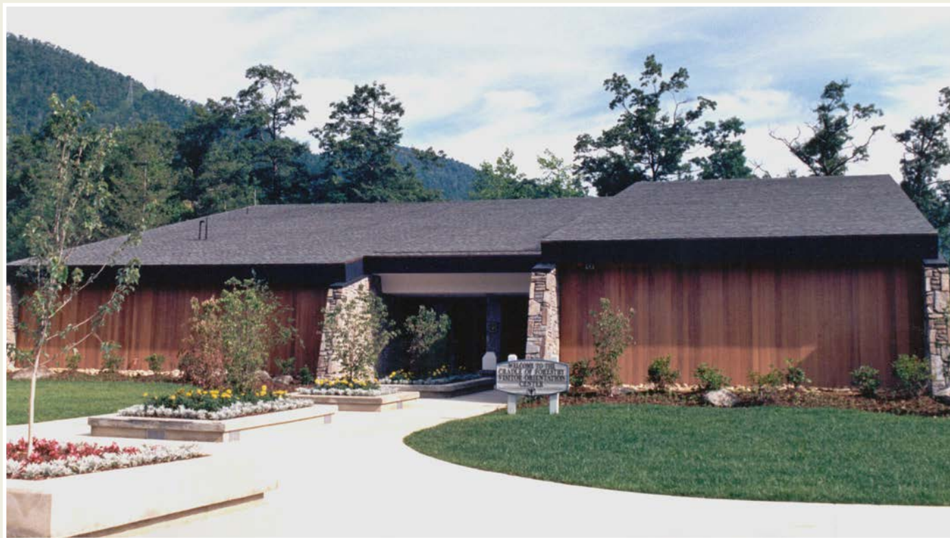
The visitor orientation center at the Cradle of Forestry in America national historic site located in the Pisgah National Forest near Asheville, North Carolina, in 1988. From here it is a short walk to a reproduction of the schoolhouse.
