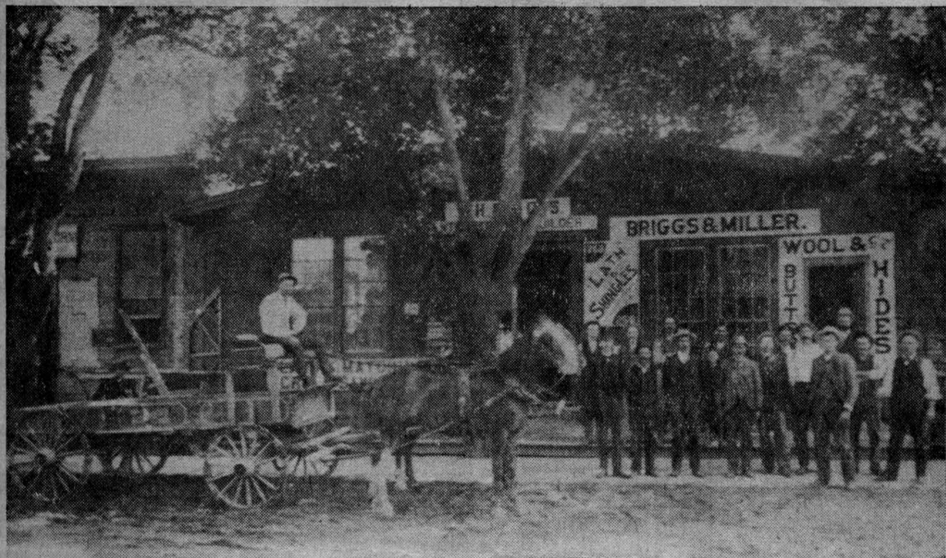
OLDEN DAYS —The 60 year old Briggs Lumber Co. began in the shade of Main Street on the present site of the postoffice. Since then, the business has expanded to nine branches including the new yard acquired in Dimmock, Pa.
