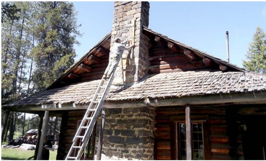
Students from Eastern Oregon University and Clatsop Community College documented and measured the log building before its disassembly in 2015.
