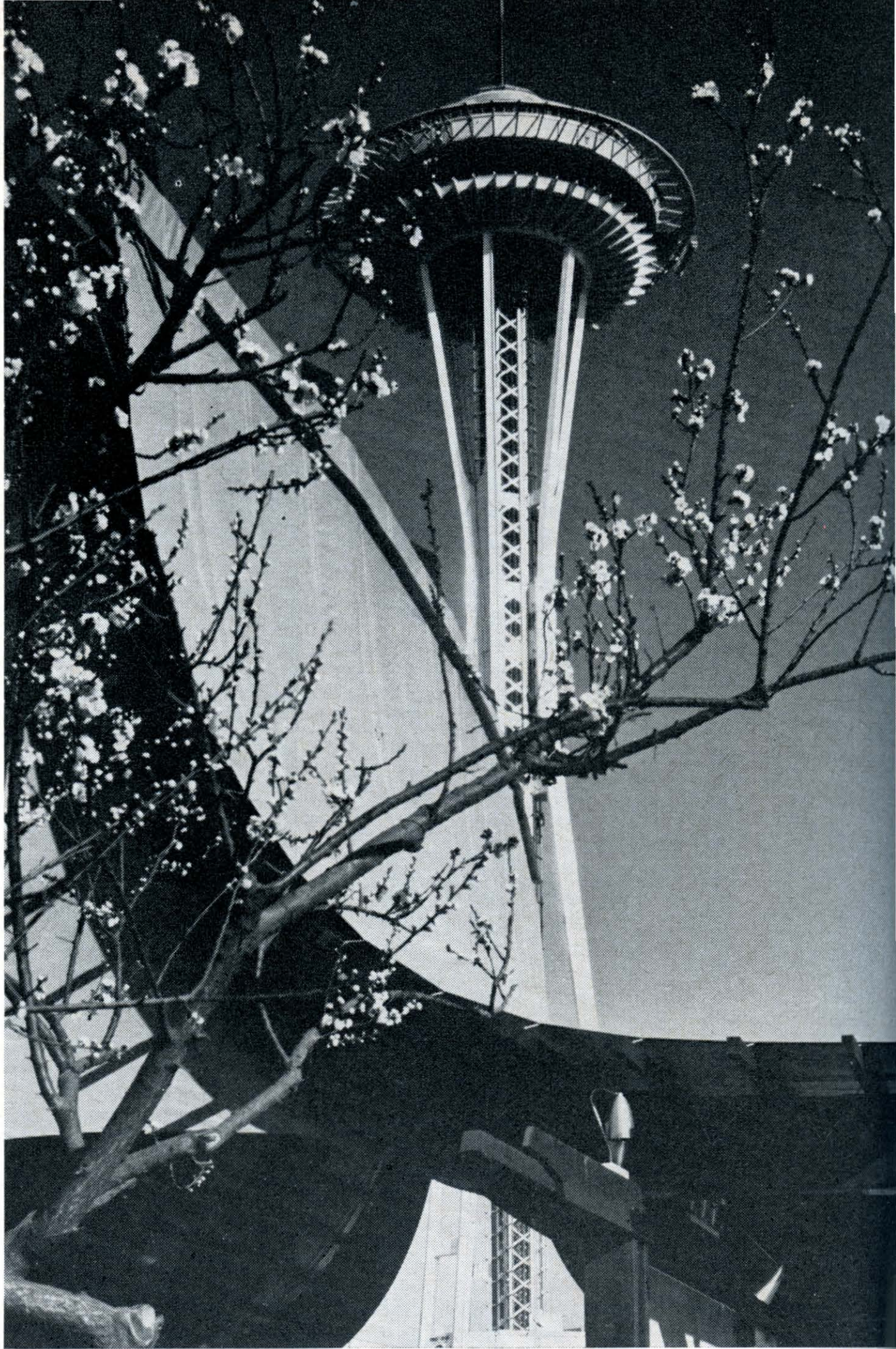
The Space Needle, with its rotating restaurant on top, towers above General Insurance Company's Information Center with its graceful Douglasfir glued laminated arches—30,000 boardfeet of lumber, plywood, and wood products
