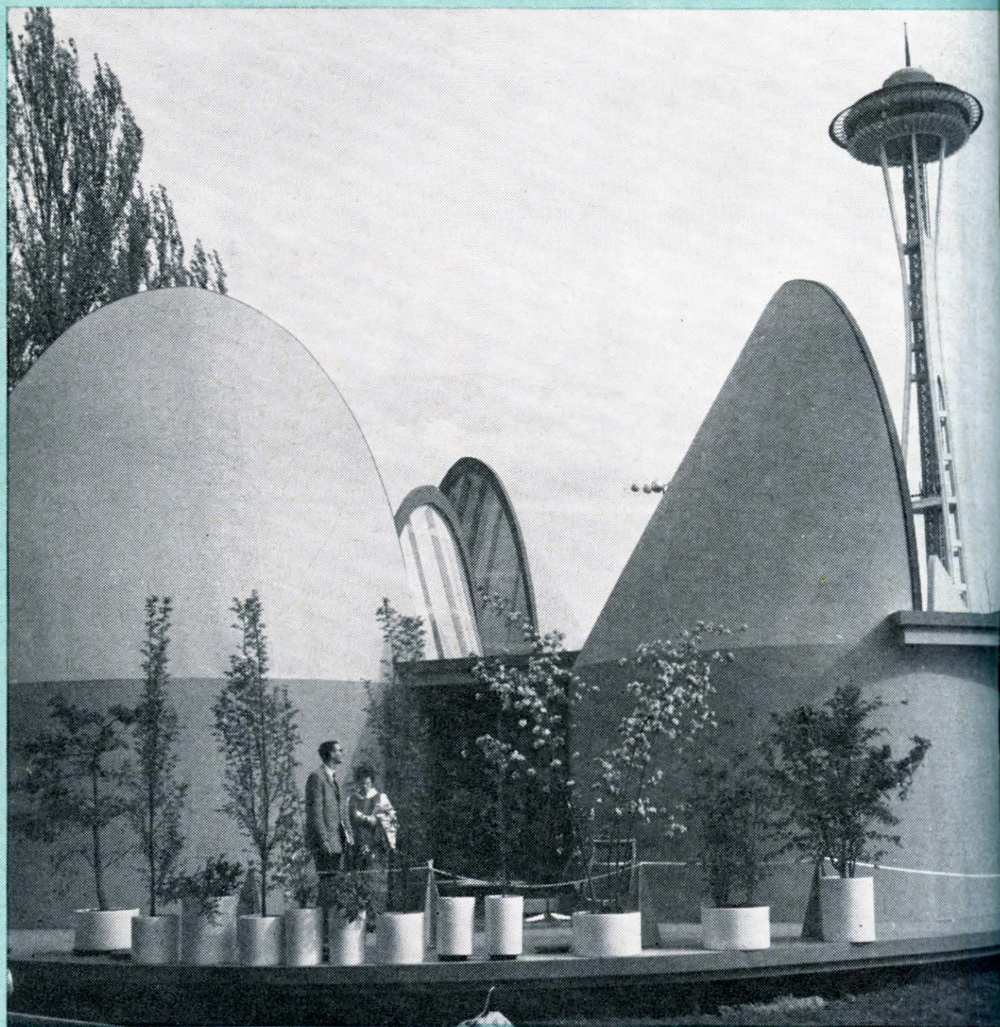
“Plywood Home of Living Light” has as its most striking features six hemi-paraboloid domes of molded plywood and transparent acrylic plastic. These skylights rotate on circular tracks to follow the sun and provide shadow-free north lighting all day
