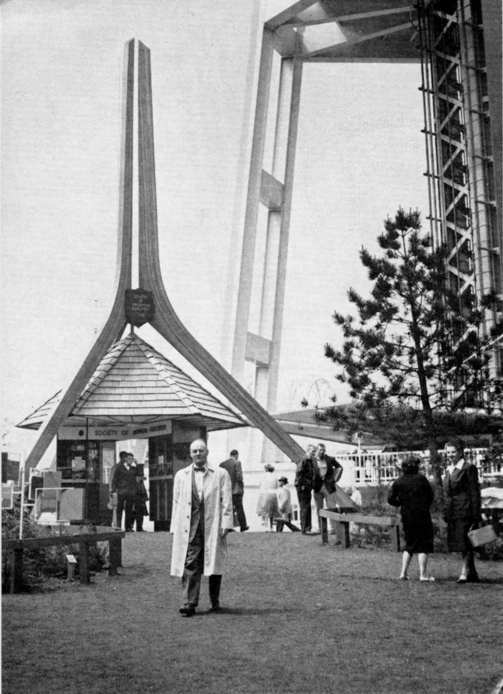
SAF exhibit area provided a green oasis amidst World Fair acres of concrete and asphalt. Seven islands of trees dotted the area and benches were provided for weary fairgoers. Behind information booth can be seen steel leg of 600-ft. high Space Needle.
