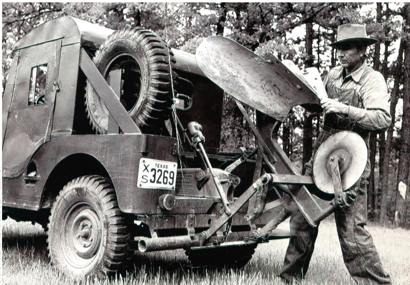
A fire plow attached to a World War II surplus military jeep was used by TFS crews to build fire breaks in the 1940s.
