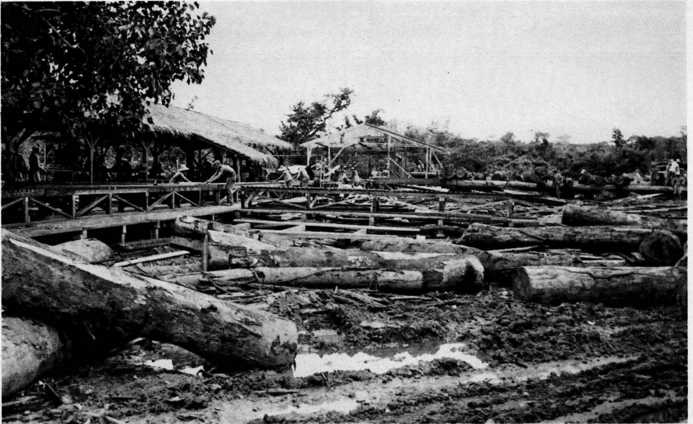
The sawmill setting of the 1002nd Engineer Forestry Battalion is located on the very road over which the infamous "death march" of Bataan took place in 1942. Logs came in by truck and tractor. Note the extensive use of gravity rolls for handling lumber. An everlasting struggle with mud was fought in the woods and around the mill yard.
