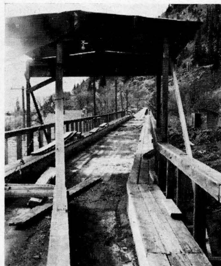
Flume terminal at planing mill, where V-section gives way to flat channel. (Shown dry during repair operations.)
