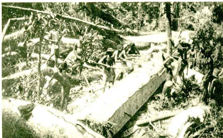
"SQUARING" MAHOGANY LOGS IN THE BUSH THE MAN AT THE LEFT WITH THE TWO "MACHETES" IS BEATING THE TIME AND THE MEN ON OPPOSITE SIDES OF THE LOG ARE SUPPOSED TO WORK IN UNISON
