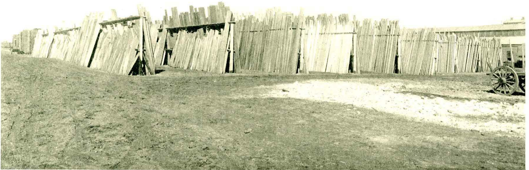
THE "SUNNING RACKS"—CAPACITY A MILLION FEET ASSURING WELL COLORED MAHOGANY.
