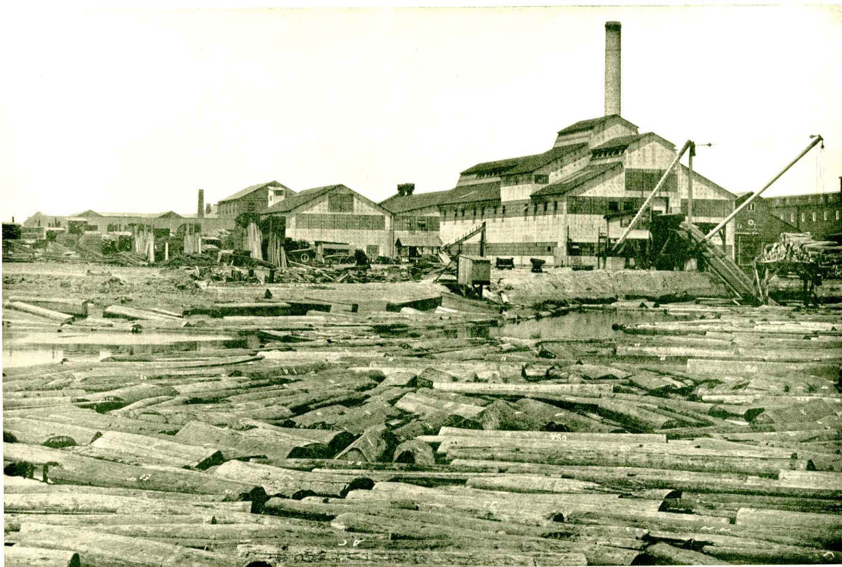
SAW MILL—SHOWING “FEEDING NECK” OF LOG POND. ( Extension, left center, is exterior of lumber inspection room. )
