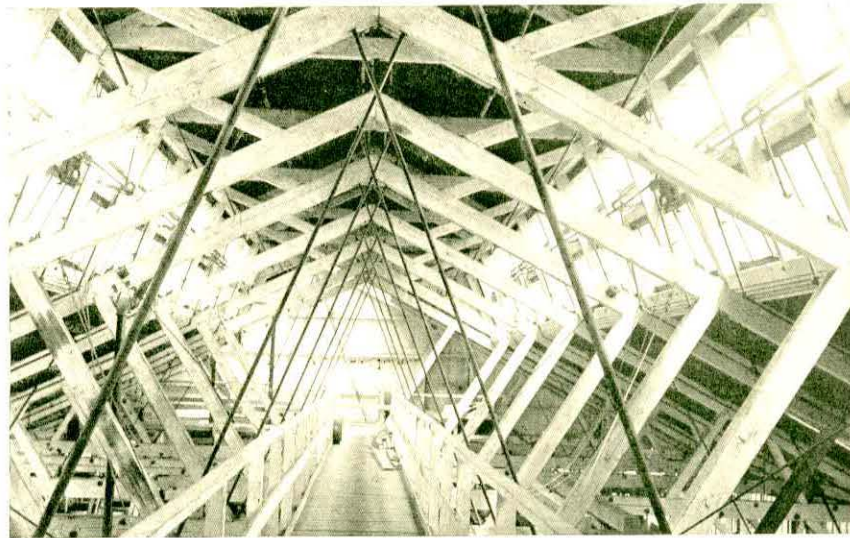
WALK ABOVE MILL FLOOR—SHOWING TRUSS CONSTRUCTION
