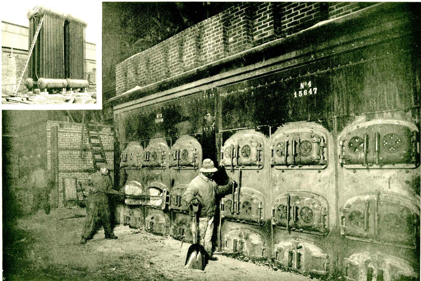
"BABCOCK & WILCOX"—WATER TUBE BOILERS ( Rust-type ) THREE WITH "DUTCH-OVENS"—CONVEYOR FEED. Insert— NO. 3 & NO. 4 DURING ERECTION.
