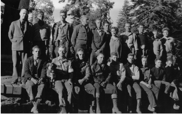
"The gang ready for work on the Robbs Peak project, California, 1937. On Georgetown Ditch bridge." Evans is presumed standing at the far left end. (FHS8399)
