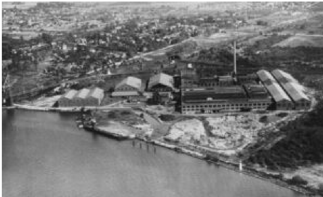
Aerial photo of the Kieckhefer Container Plant in Plymouth, 1962.
