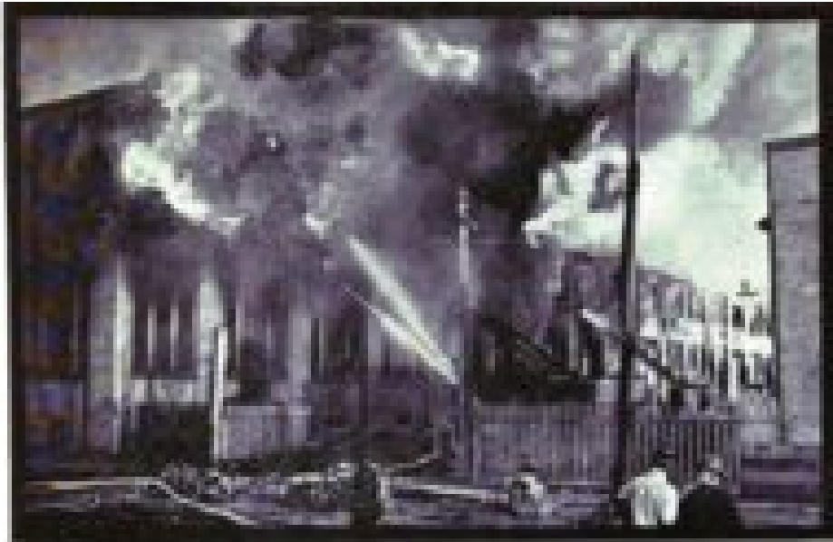
Upper Picture Shows Great Crowd Gathered on Sixteenth Street While Staff Watching Fire—Lower Picture Shows Burning Plant.
