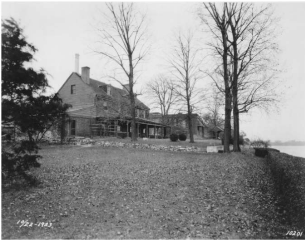
Old Isaac Fish Homestead, the new office for the Kieckhefer Container Company.
