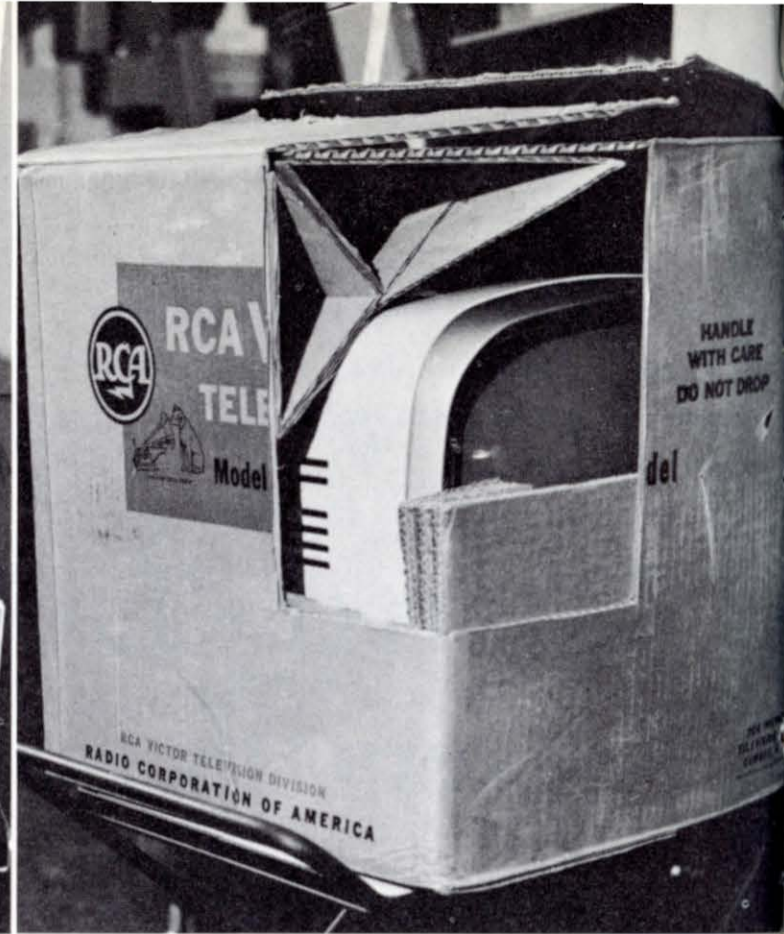
CUTAWAY CARTON for TV set shipment shows intricate and sturdy packaging that ensures the product's arrival in undamaged condition.
