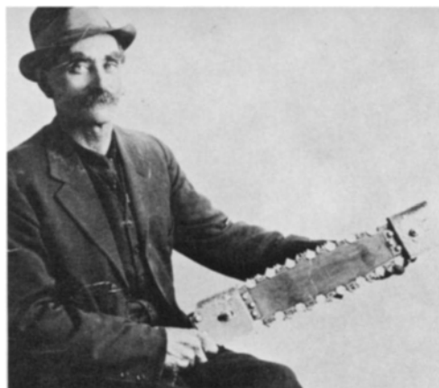
There were numerous experiments with power saws. James Shand, a Manitoba farmer and millwright, patented his "endless chain" saw in 1918 and took a gasoline-powered model to British Columbia, hoping to interest the lumber industry in its production. Failing to do so, Shand allowed his patent rights to lapse in 1930.
