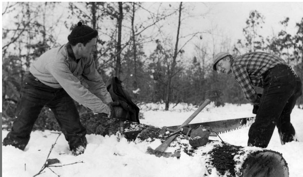
Dick Mommsen and Lloyd Hulbert sawing out ties from a recently felled tree in February 1943. Note that the snow is up to the men’s knees.
