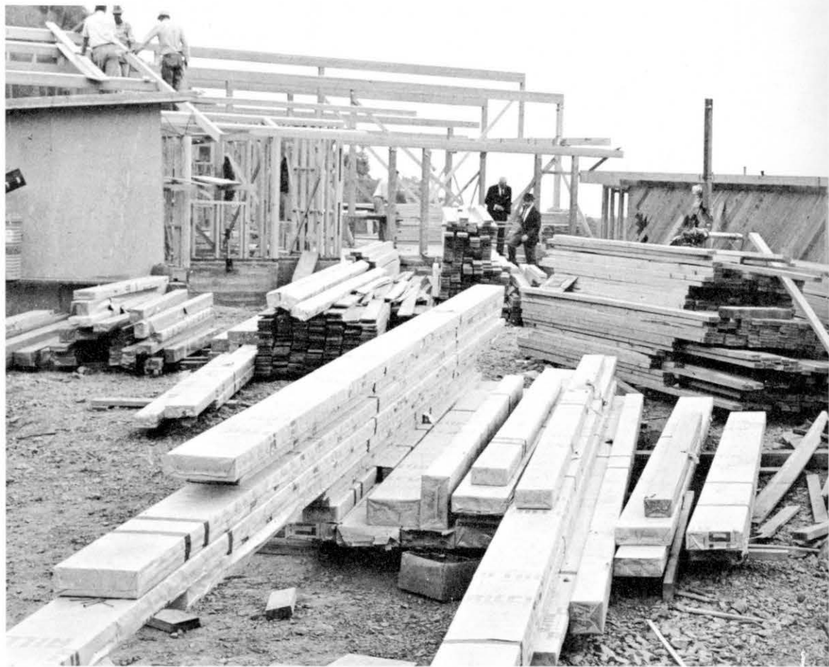
WEYERHAEUSER LUMBER products are stacked on the job site. In the foreground are Rilco Laminated Rafters which support fir roof decking.
