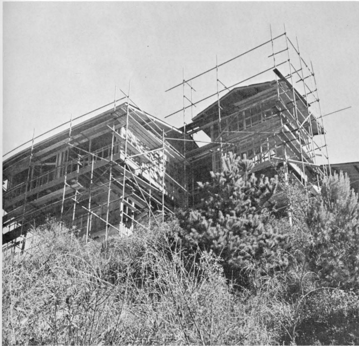
STRIKING MOVIE HOME perches half-way up a 130-foot steep hillside lot with a spectacular view down a canyon to the Pacific Ocean. For maximum strength, rigidity and wind, the design called for kiln-dried structural lumber throughout and diagonal wood sheathing on certain walls.
