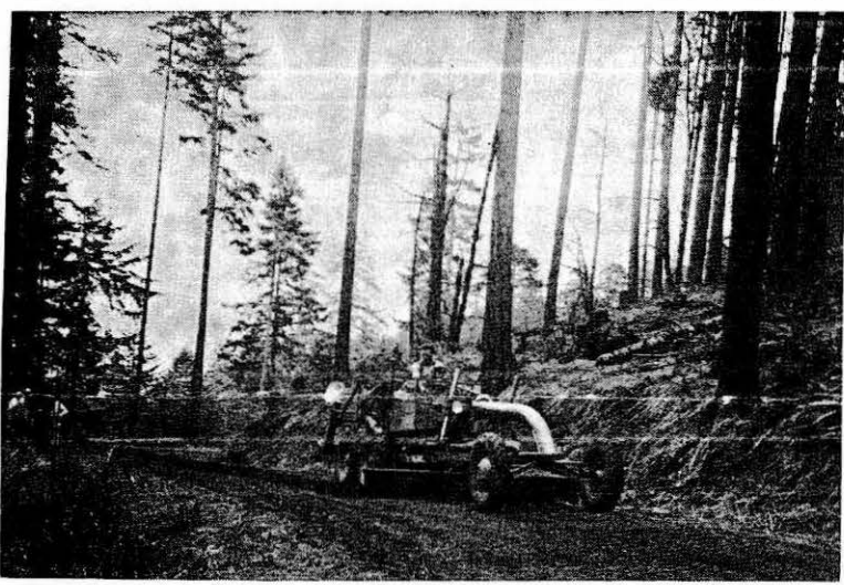
An important part of the Oregon State University School of Forestry operations, logging roads are kept in top condition the year 'round by an Allis-Chalmers model D motor grader.
