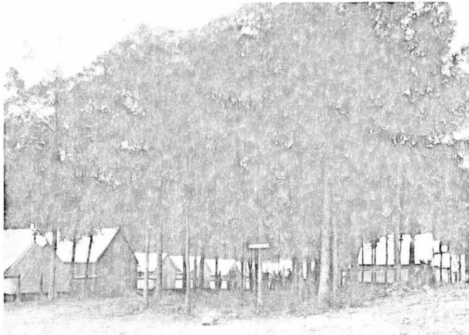
With 25,000 unemployed men already in conditioning camps, preparatory to work in the forests, camps similar to the one pictured above are rising in many forest regions. In these comfortable and healthful tent cities, equipped to take care of as many as two hundred men and more, the conservation corps will be quartered.
