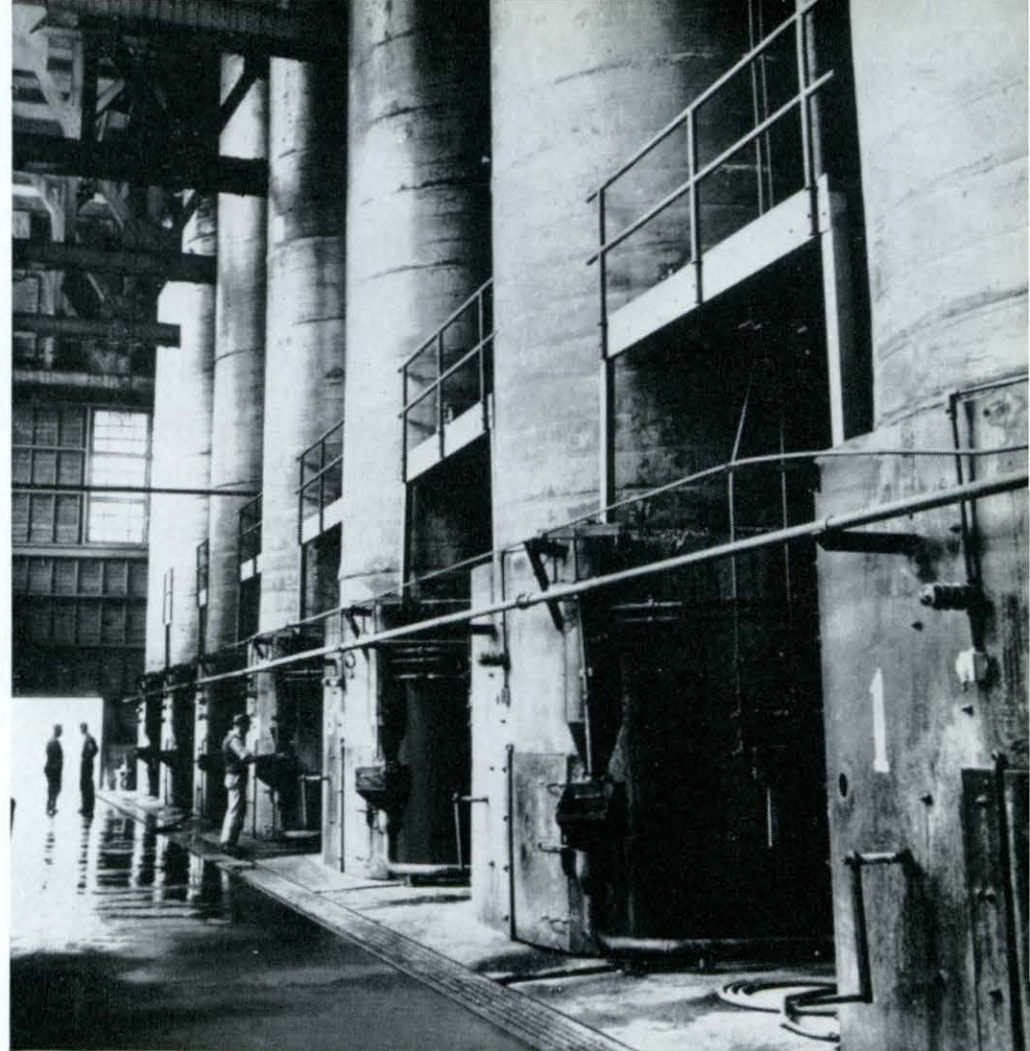
Chips are cooked in these huge digesters until reduced to wood pulp.
