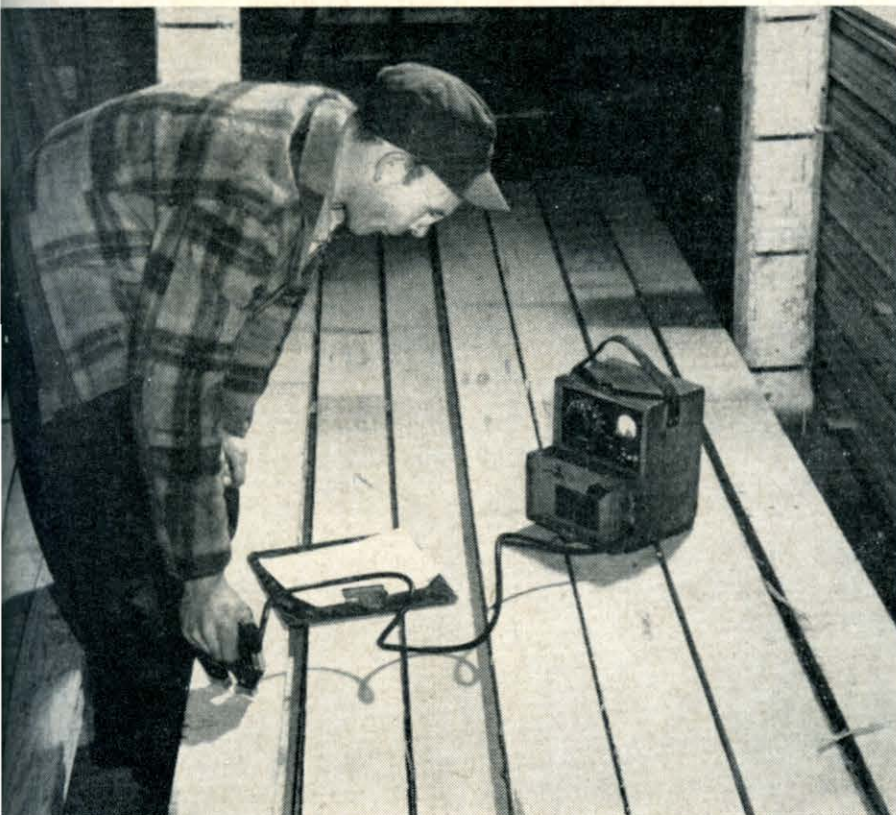
One of the newer mechanical aids for testing lumber quality is device which registers moisture content
