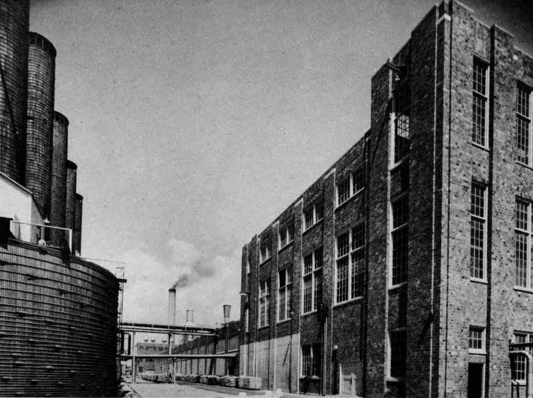
The pulp screen room, at right in the foreground, is connected by pipeline with the blow pits.
