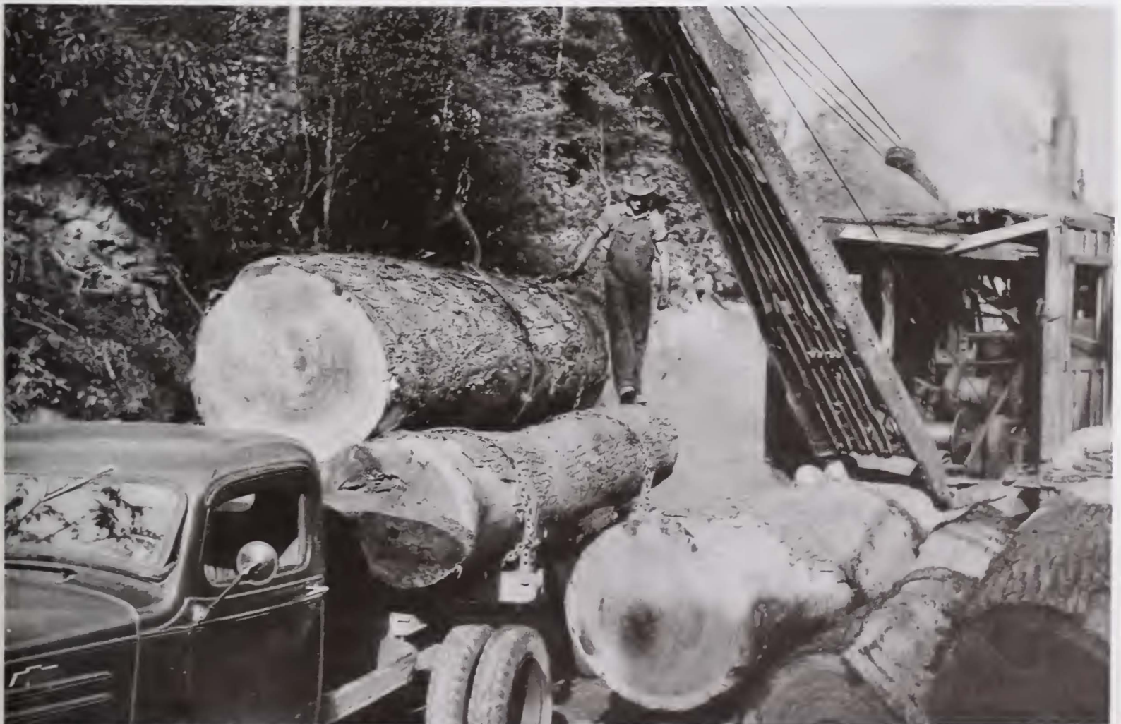
Figure 42.—Loading logs onto a truck from a roadside skidway with a steam-powered rig on rails. Spot was along the Upper Tellico River, Monroe County, Tenn., south of Great Smoky Mountains National Park, on the Cherokee National Forest, in 1937. (National Archives: Record Group 95G-354360)
