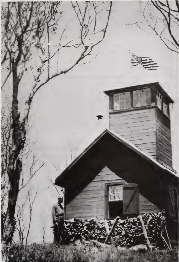
Figure 71.—Hayes Lookout, Nantahala National Forest, N.C., a low wooden enclosed structure with a 6- x 6-foot cabin, built by Civilian Conservation Corps enrollees in 1939. (NA:95G-396050)
