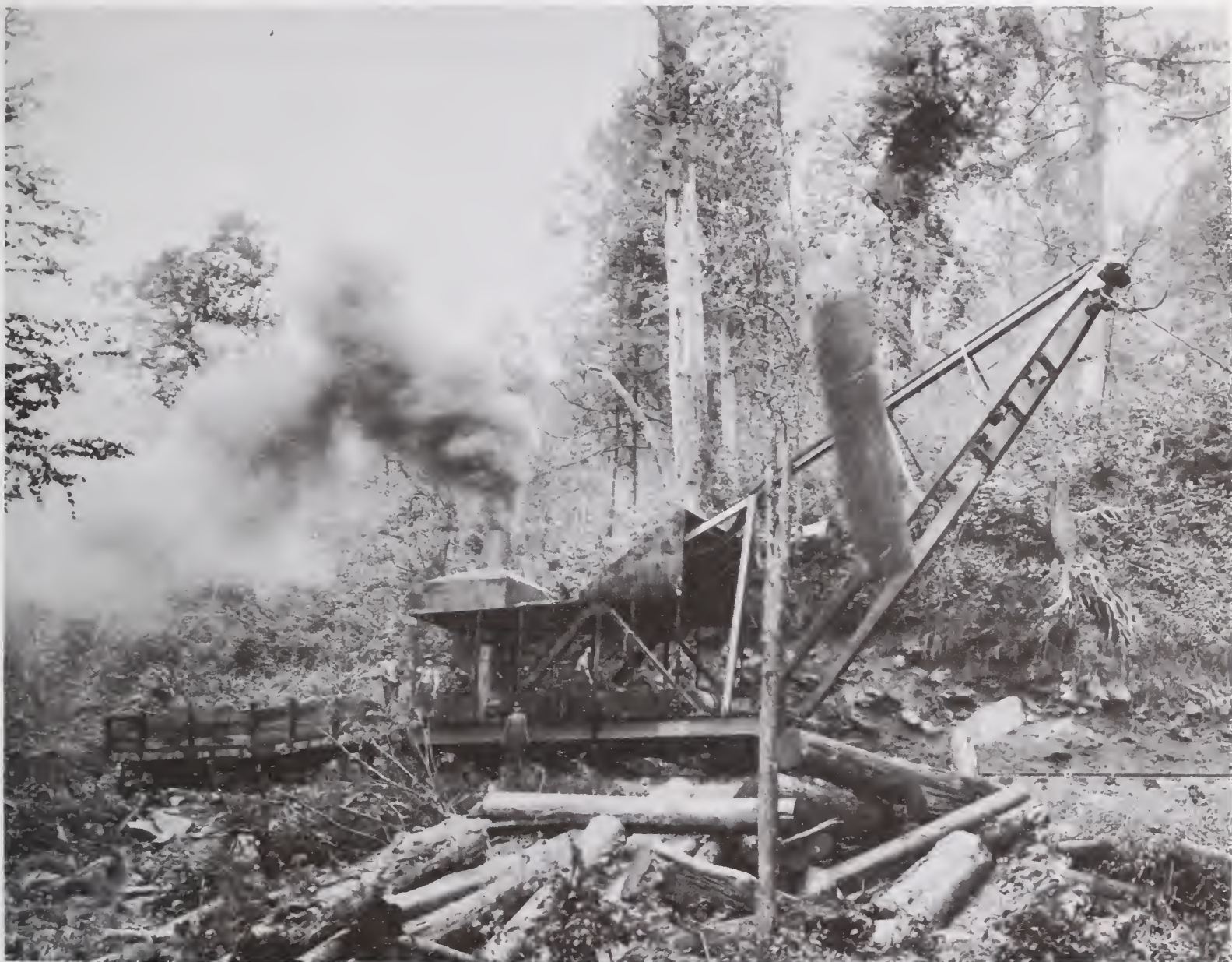
Figure 15.—Steam overhead cable skidder on rails bringing in logs from two facing slopes on tract of Little River Lumber Company in Great Smoky Mountains, Sevier County, Tenn., in 1913. (NA:95G-15507A)
