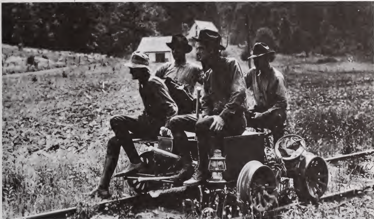
Figure 36.—Four-man crew on way to forest fire on railroad handcar, with various hand tools including pulaski, axes, pitchforks, canvas bucket, and lantern. Pisgah National Forest, N.C., 1923. (NA:95G-176444)
