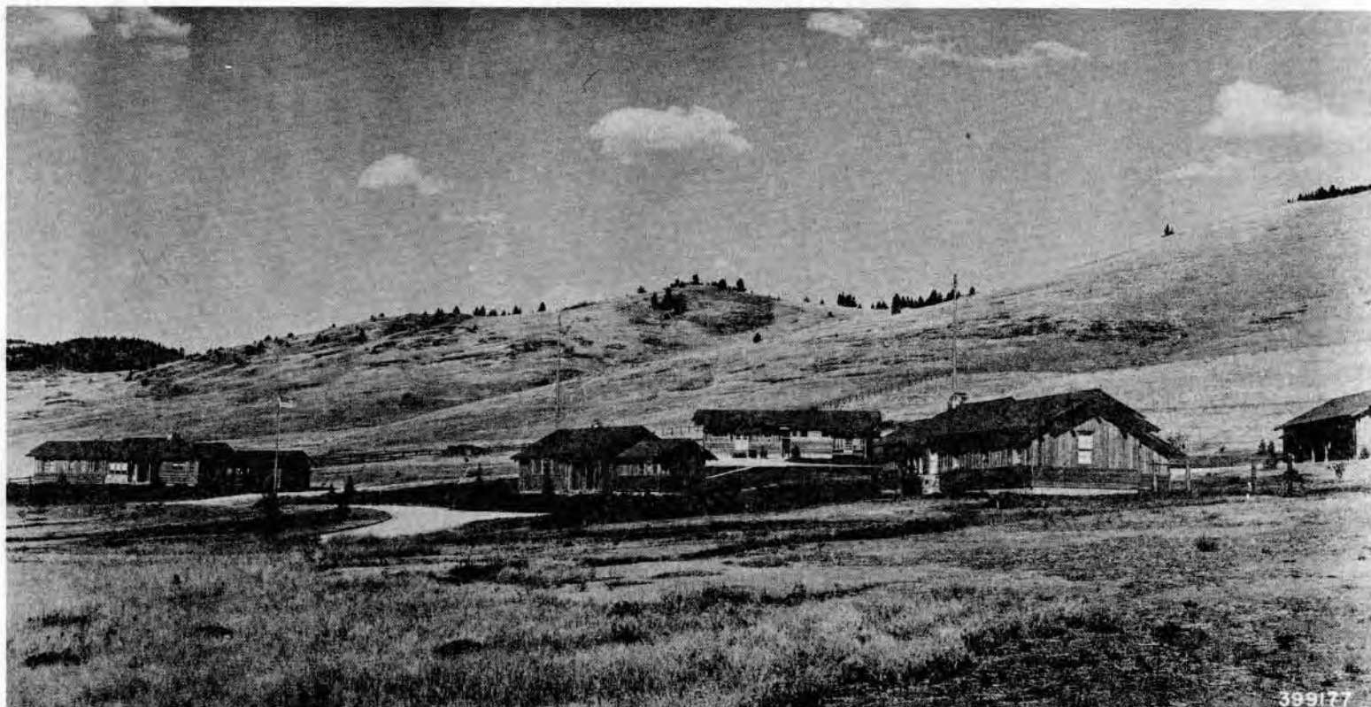
Deerlodge NF - View from SW of Philipsburg Ranger Station, built 1939. Left to right, Alternate Ranger house, administrative building, warehouse-cook and bunkhouse dwellings and shop-garage building.
