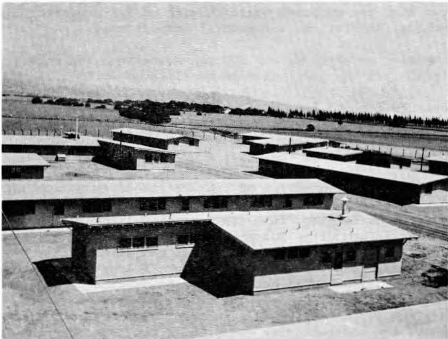
General view of labor camp built and maintained by the project for workers.
