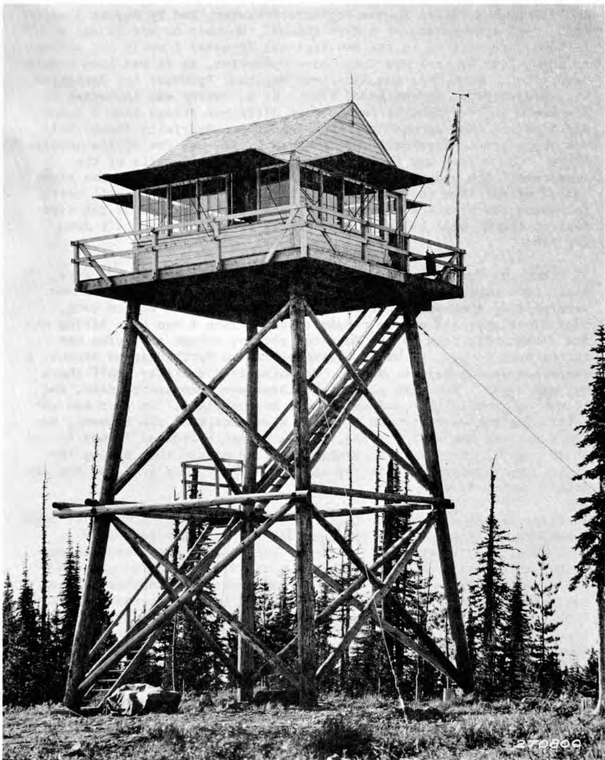
Chewelah Mountain Lookout Tower, Colville National Forest. "Readicut" in Spokane Warehouse, cargoed for mule transport, the tower was designed by C. P. Fickes in 1929.
