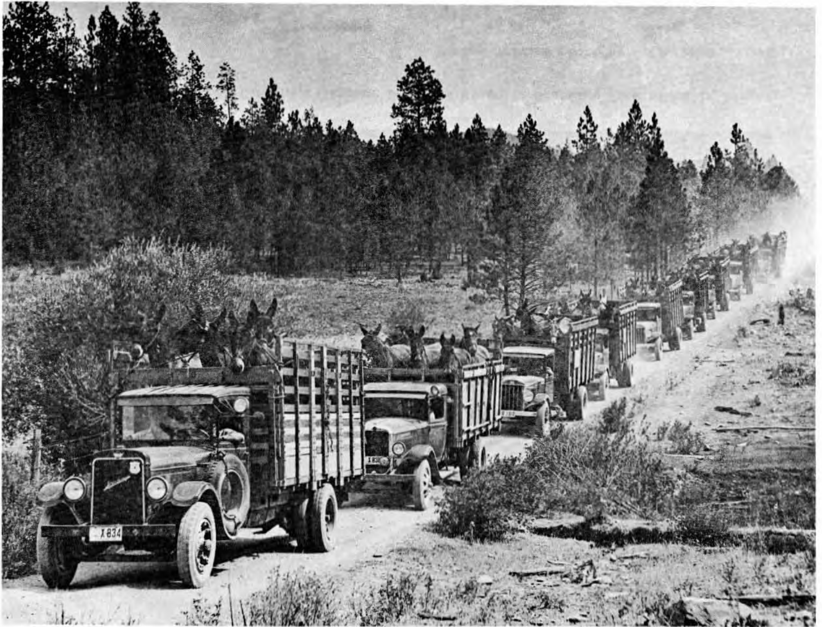
Pack strings being trucked to fire, about 1931.
