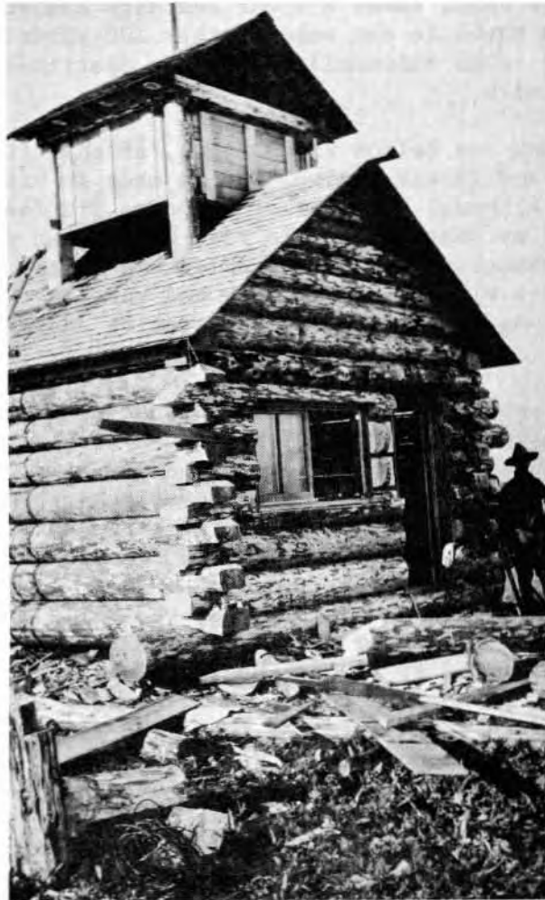
Graves Peak L0 under construction. 1920. Bill Deasy, Forest Ranger.
