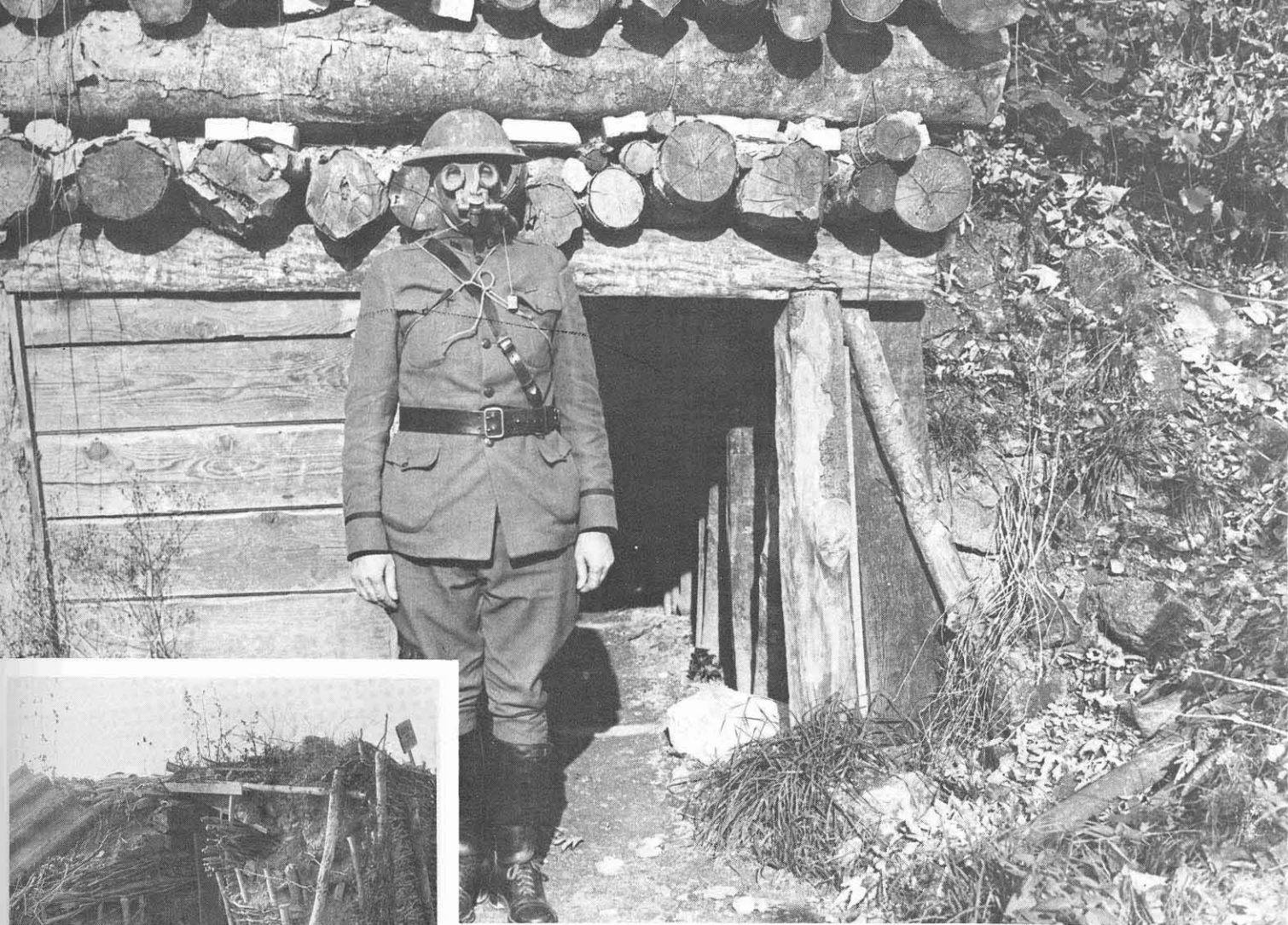
A typical American dugout along the Western Front used much wood. An army chaplain, wearing a gas mask, poses at Verdun, November 4, 1918. Inset: Branch and brush revetments.
