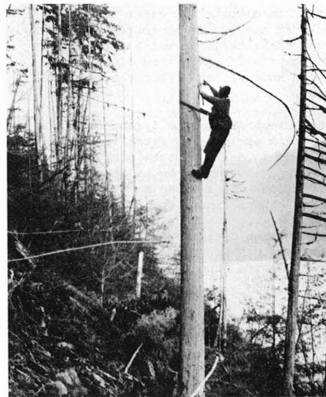
Figure 4. Ranger hanging telephone insulators on a dead tree, Olympic National Forest, Wash., April 1921. (NA:95G-157284)
