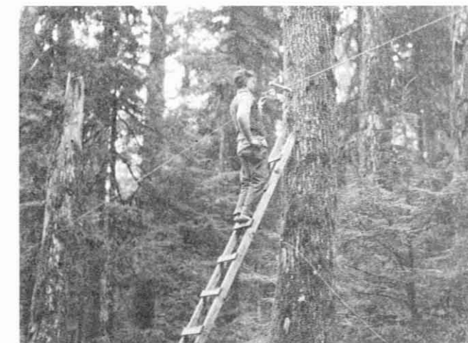
Figure 9. Wooden bracket for Forest Service field telephone lines, designed by Clay M. Allen, Pacific Northwest District (now Region) telephone engineer, to hold the wire away from the trees and thus prevent leakage of current, which would be extensive in the wet weather so common on the west side of the Cascade Mountains in that Region. 1921 photo. (NA:95G-158323)
