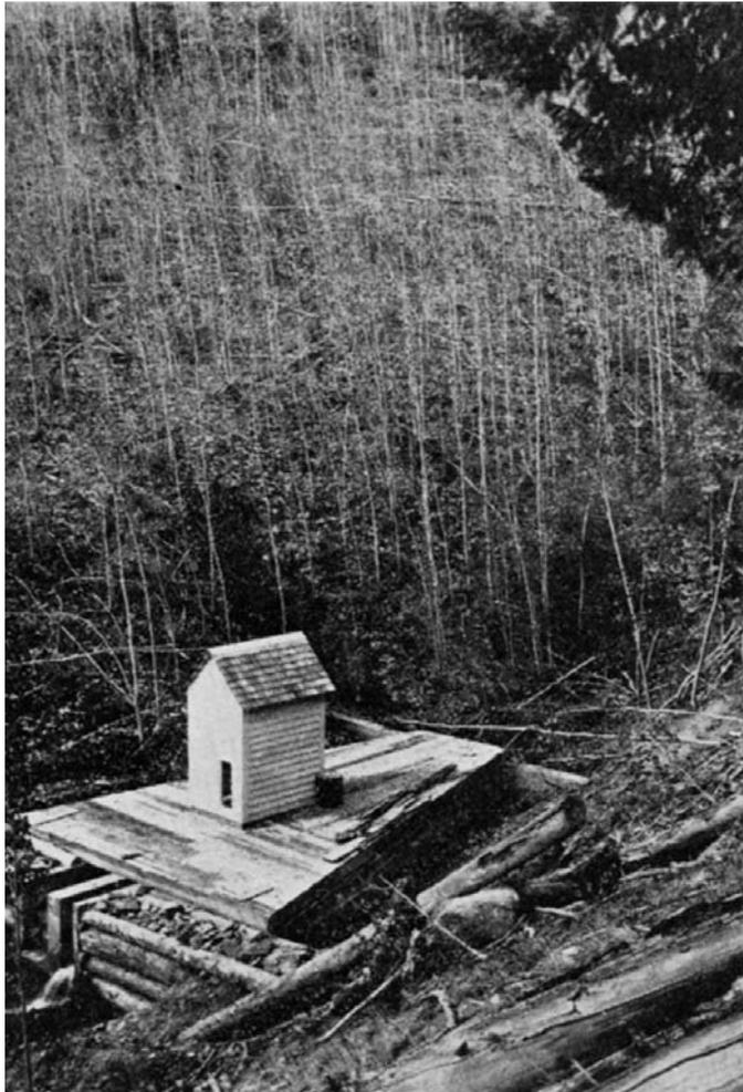
*Gaging station at Wagon Wheel Gap, Colorado. This was the prototype for later small forest watershed studies in the United States, with a control watershed and calibration period prior to treatment. USDA Weather Bureau photo (1928).*
