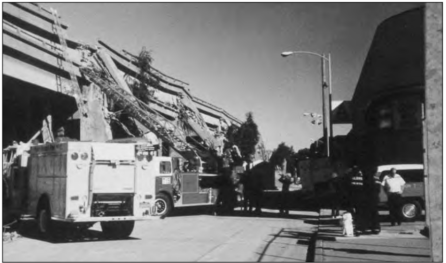
Freeway collapse in Oakland, California resulting from 1989 Loma Prieta earthquake.
