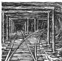
Supporting timbers and ties are used in mines.
