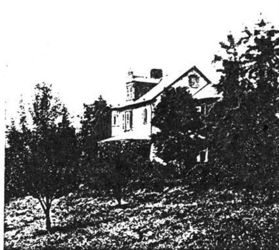
THE BUILDING OF THE YALE SUMMER SCHOOL OF FORESTRY AT GREY TOWERS, PA.
