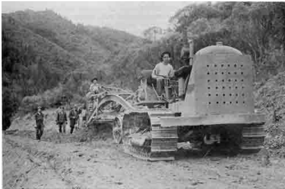
CCC enrollees operating tractor and grader on road construction. Cat Skinner, Puss Young, CCC. Bill Jones, R.R. Forest Construction Superintendent and Everett Rawlings, CCC Foreman, directly behind grader wheel. 65 Gas Cat, Applegate Camp, Austin Western Grader, Tallowbox Lookout Road via Star Gulch.
