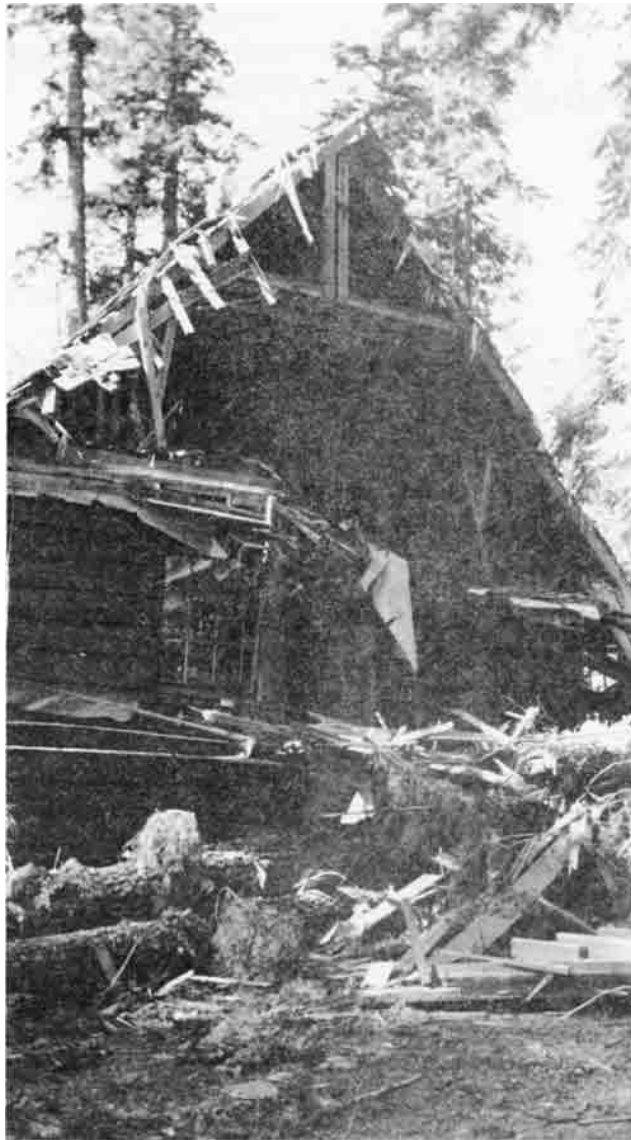
Lake of the Woods warehouse damaged by Douglas-fir windthrow.
