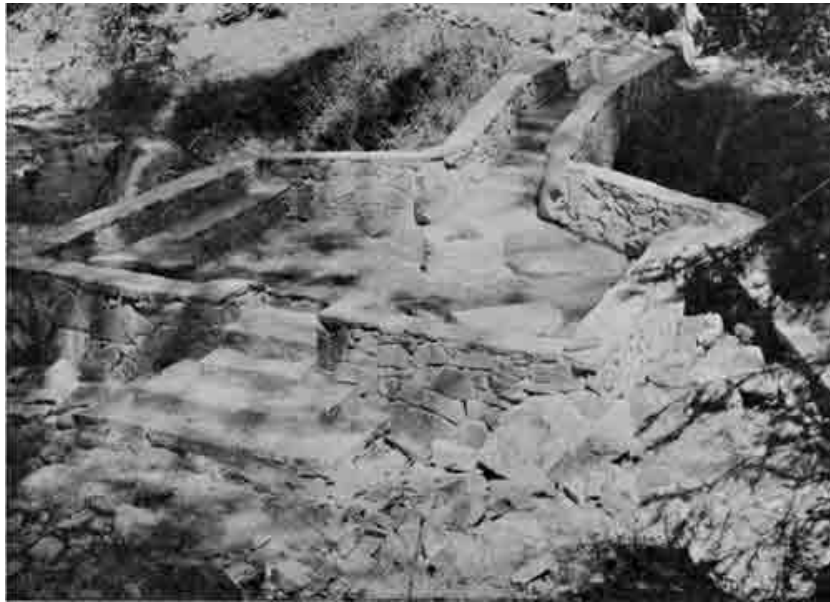
This is a cleanup of the spring enclosure and bridge shown above. This structure was washed out in the Dec. 1964 storm and floods.
