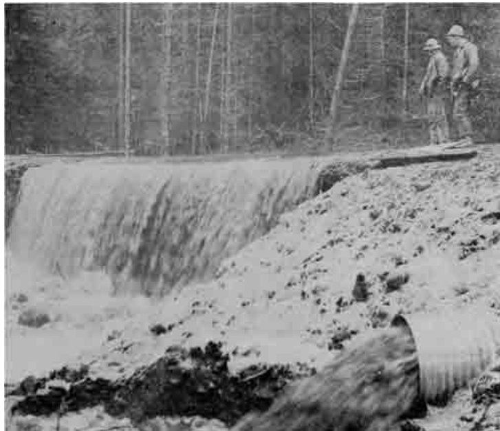
Photo of water scour across Parsnip Creek Road #344C from Titanic Creek. This picture was taken before the road was breached. Note the complete utilization of the culvert by flood waters.
