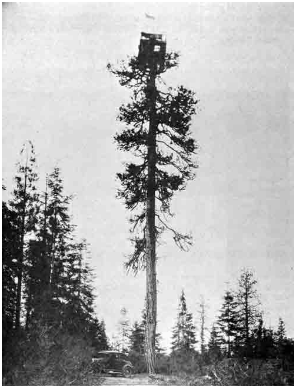
Inexpensive lookout tower on Agency Butte 106 feet from ground to fire-finder. Tree is a western yellow pine. Iron pins. - L. D. Bailey, 1930
