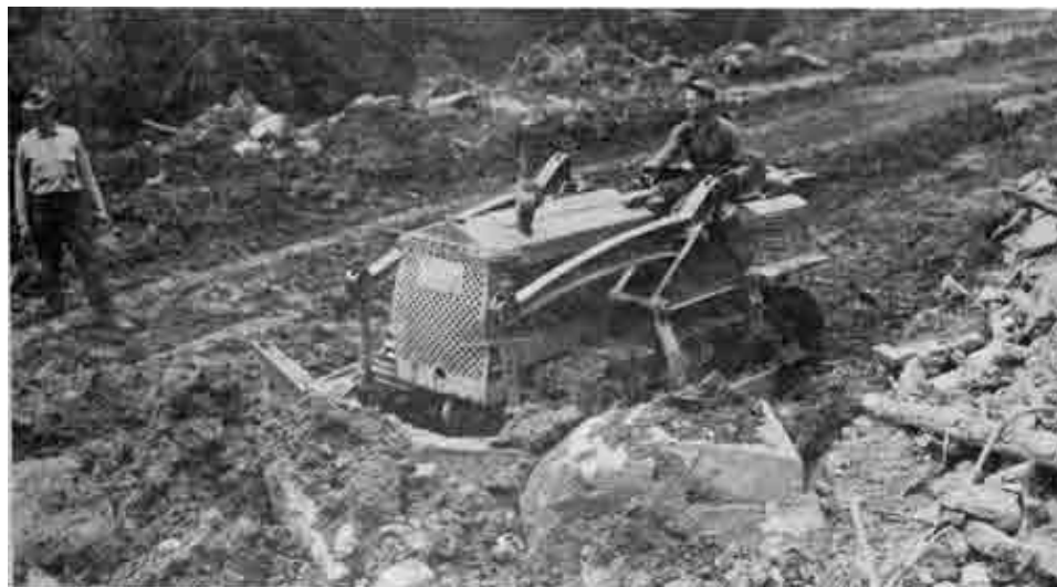
CCC enrollee operating Cletrac "55" tractor on road construction.
