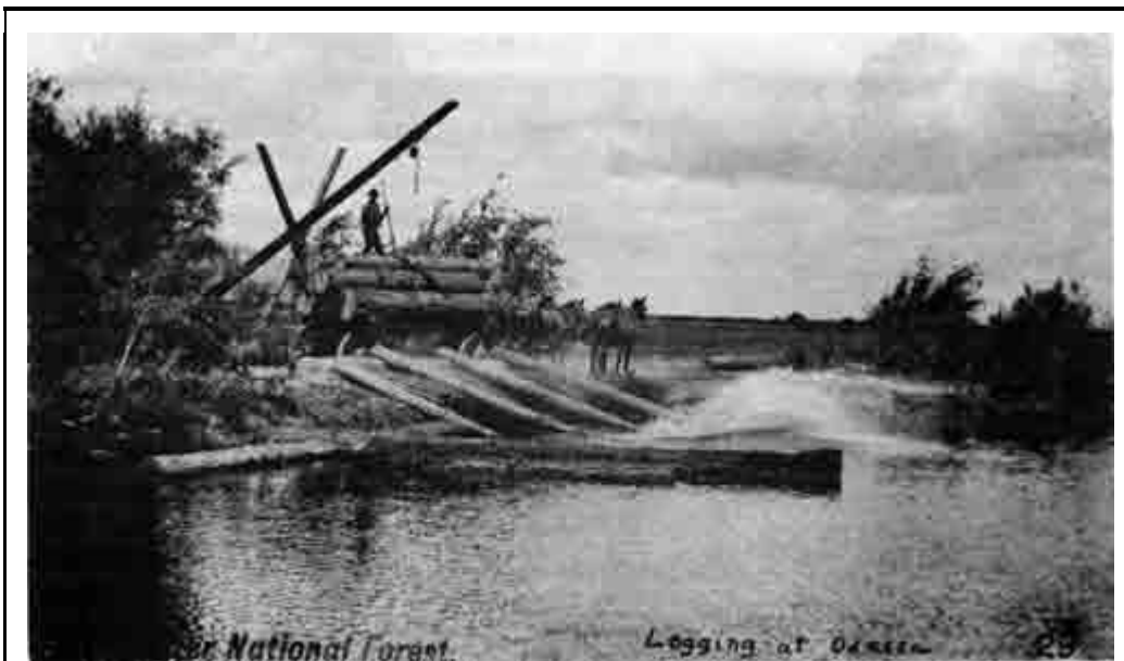
Unloading logs at Odessa on Klamath Lake, 1908.
