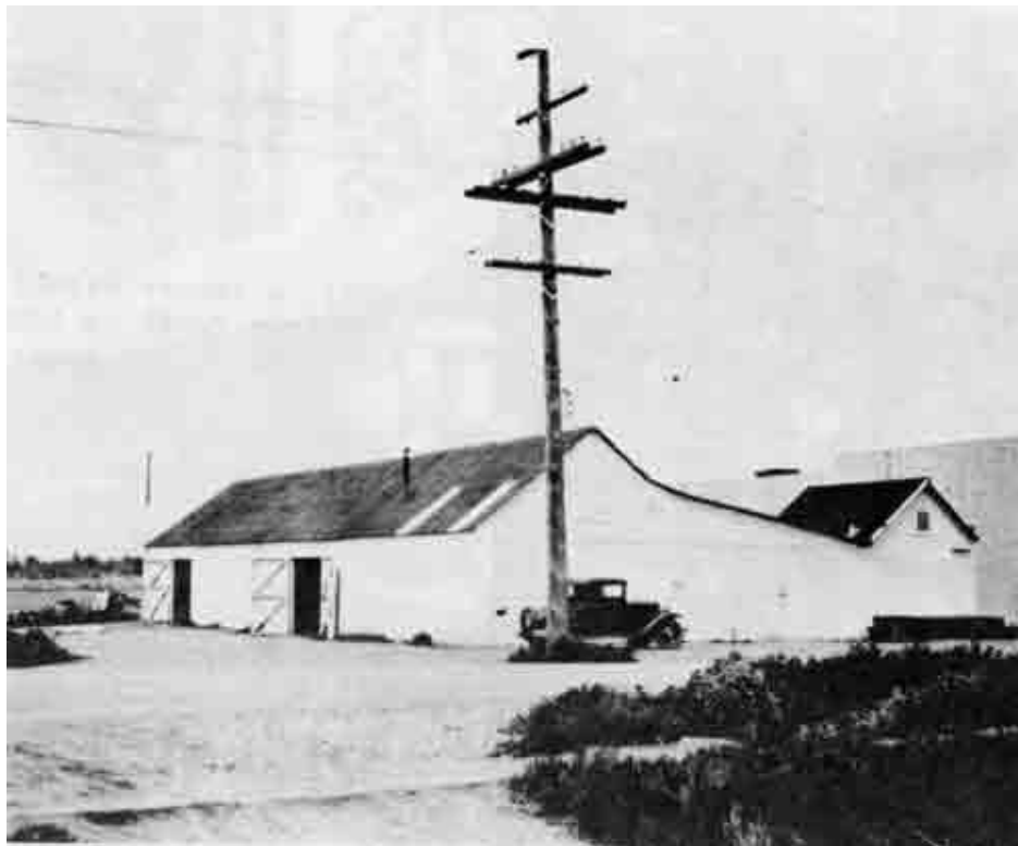
Forest Service Warehouse and Shop, Medford, Oregon built in 1925 and '26 near Jackson and Hawthorne Streets. - Lee P. Brown, May 13, 1927
