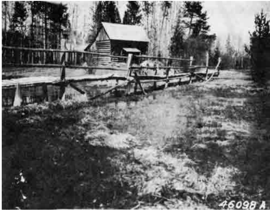
Pelican Ranger Station - H. D. Foster, 1910
