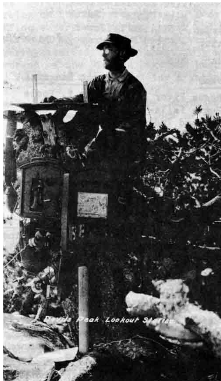
Devil's Peak Lookout Station. Iron Mine telephone and a crude temporary alidade whittled from shakes. - E. W. Smith, 1915.
