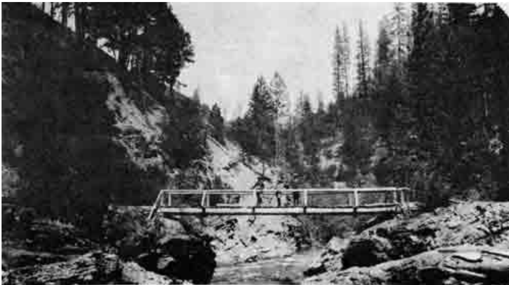
Forest Service trail and trail bridge across the Middle Fork of the Applegate River. Used by stockmen and miners in their use of the forest, and by scouts, fishermen and hunters for their recreation in the forest. In the photo a group of Boy Scouts had stopped on the bridge during a hike. - I. P. Brown
