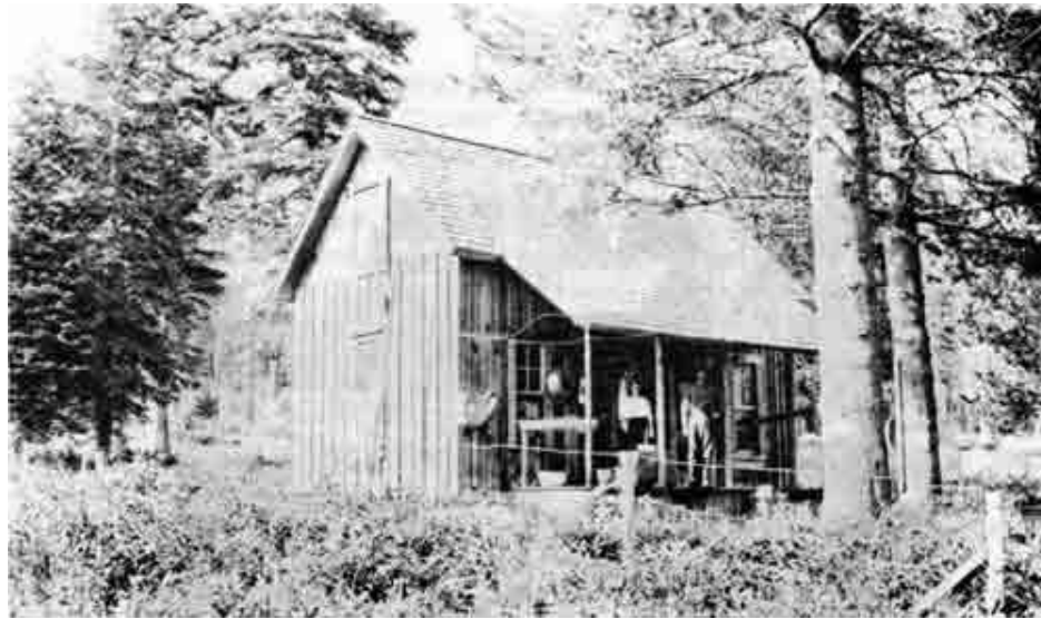
Clover Creek Ranger Station. Built by Walter and Mrs. Wright in fall of 1910; two-story house, 16' x 24'. — M. F. Patterson, 1913
