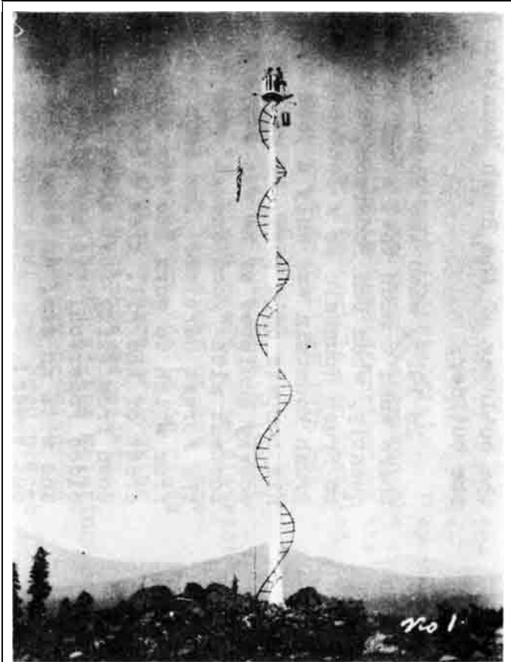
At top, lookout tree on Brush Mountain soon after construction began. The spiral ladder was 80 feet high, made of yew pegs driven one foot into the tree, with a railing of Douglas fir poles. (Photo by H. D. Foster) At bottom is shown the completed structure in 1916. Lookoutman Dan Pederson constructed the tower alone, including rigging the 5 x 5 foot square platform weighing 250 pounds, and installing the elevator (the bucket-shaped object hanging below and to the right of the platform). (Photo by A. D. Peachey)
