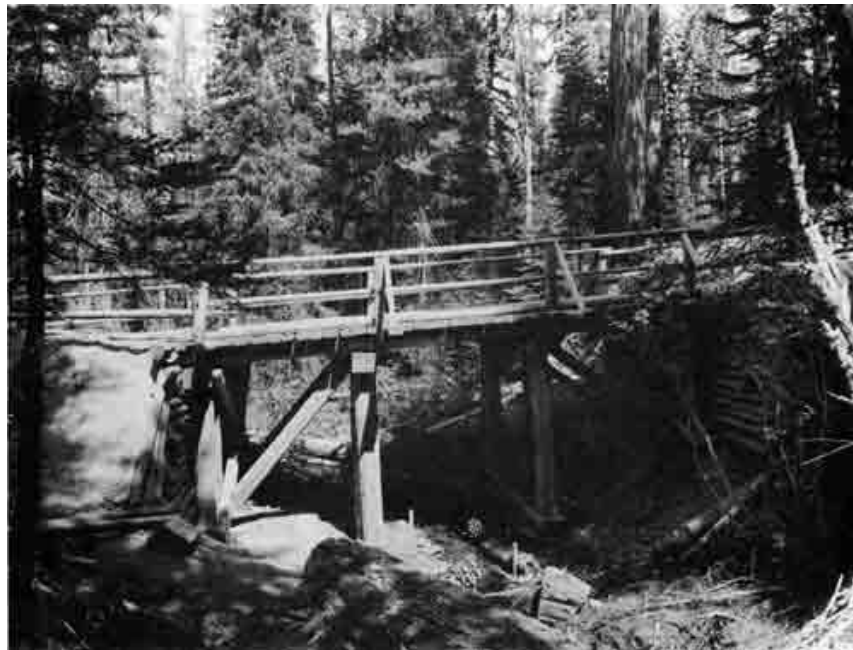
Whiskey Creek Bridge from upstream, built on Medford-Crater Lake Road in 1911 by the Forest Service at a cost of $150. - A. G. Varela, 8-29-11.
