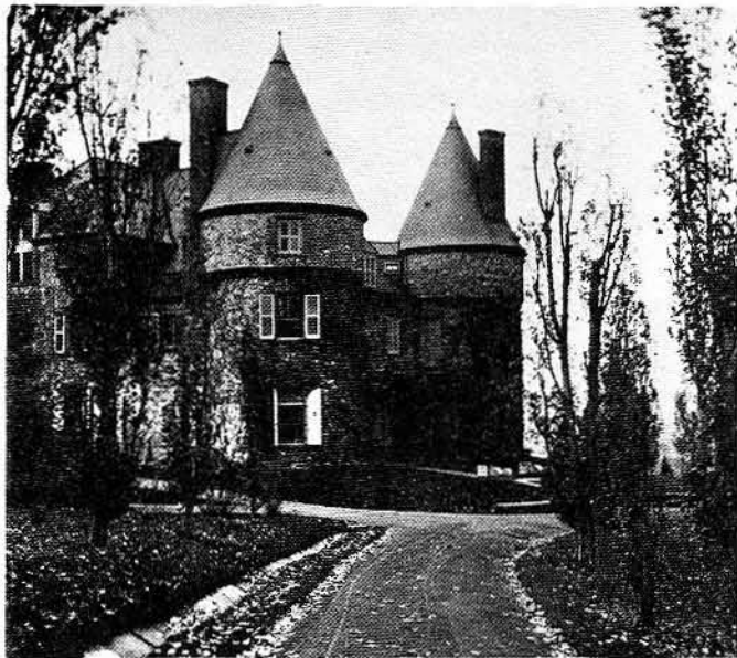
Figure 9. The main entrance facade of Grey Towers was not obscured by trees in this early view, taken from the southwest. Although the stereopticon card from which this photograph is taken was not dated, it was probably made circa 1900. From the Gifford Pinchot Papers.
