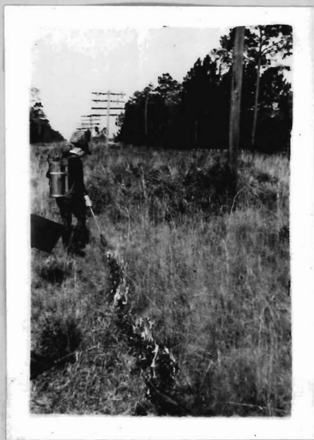
Propane torch being used in hazard burning along railroad right of way - OluStee Section-Florida National For- est - Florida.
