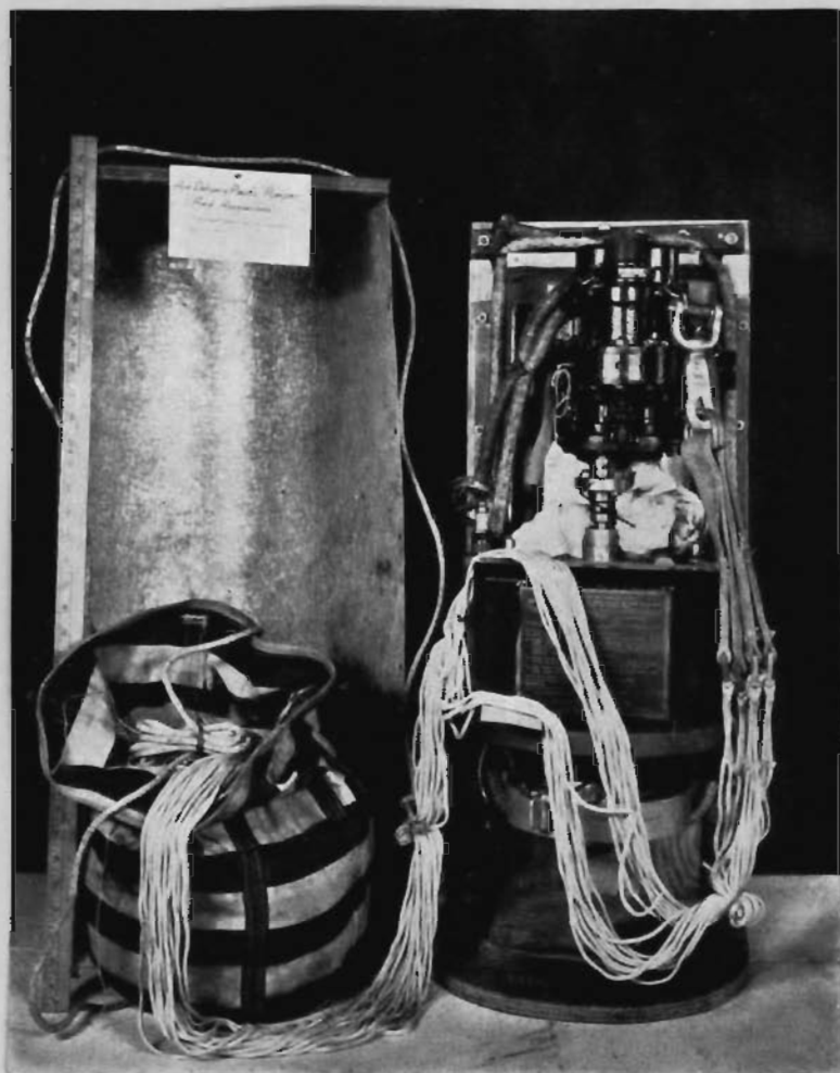
(Photo by U.S. Forest Service - Fire Equipment Handbook.) Portable power pumper, in special parachute pack, ready for aerial delivery.
