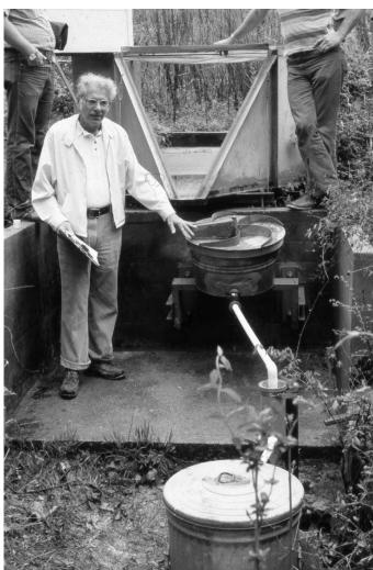
H-flumes and Coshocton wheels like this one at the Oxford, Mississippi, Hydrologic Laboratory were used in the mid-South studies to measure flow and sediment runoff from catchments with different harvesting and site preparation practices. The Coshocton wheel rotates to expose a slot that collects a fixed proportion of the flow coming off the watershed. Dr. Stan Ursic of the Hydrologic Laboratory demonstrates how the wheel works.
