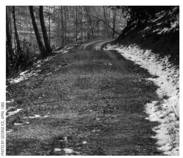
Studies on how to control road erosion were conducted at Coweeta and Fernow. This study of road erosion at Fernow, West Virginia, looks at rolling dip roads as a means of getting water off the road and minimizing erosion.
