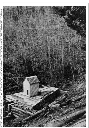
Gaging station at Wagon Wheel Gap, Colorado. This was the prototype for later small forest watershed studies in the United States, with a control watershed and calibration period prior to treatment. USDA Weather Bureau photo (1928).
