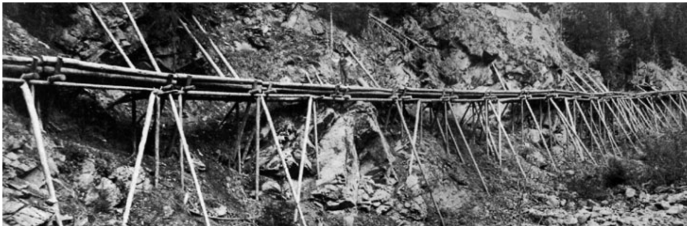
Wooden channel for timber transportation, Lower Engadin in 1886. The construction in the Schlierentäler might have looked quite similar.
