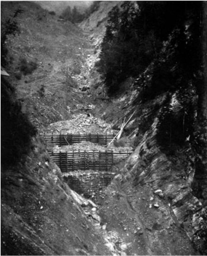
Erosion control measure on the Kleine Schliere (1880s).
