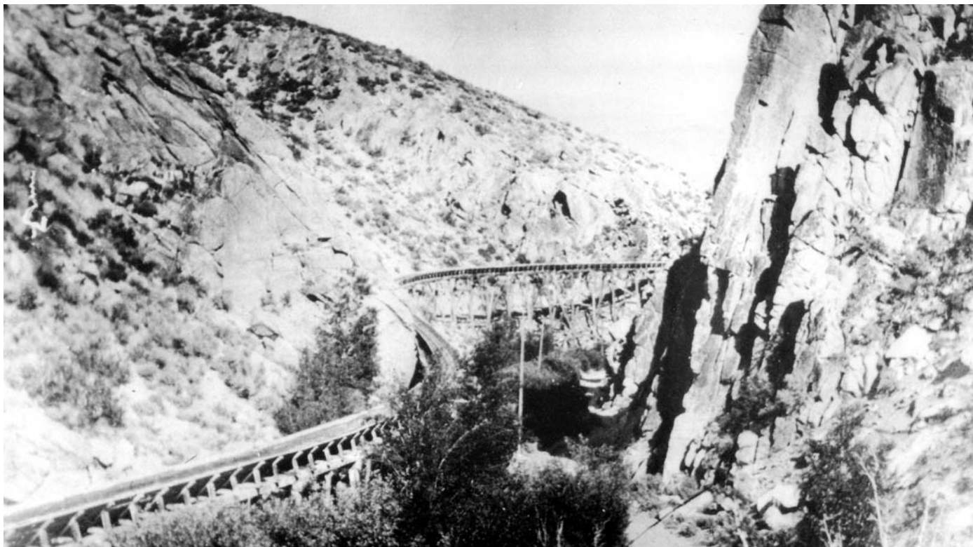
The Carson and Tahoe Lumber and Fluming Company's flume in Clear Creek Canyon. Clear Creek Road follows the old flume route.
