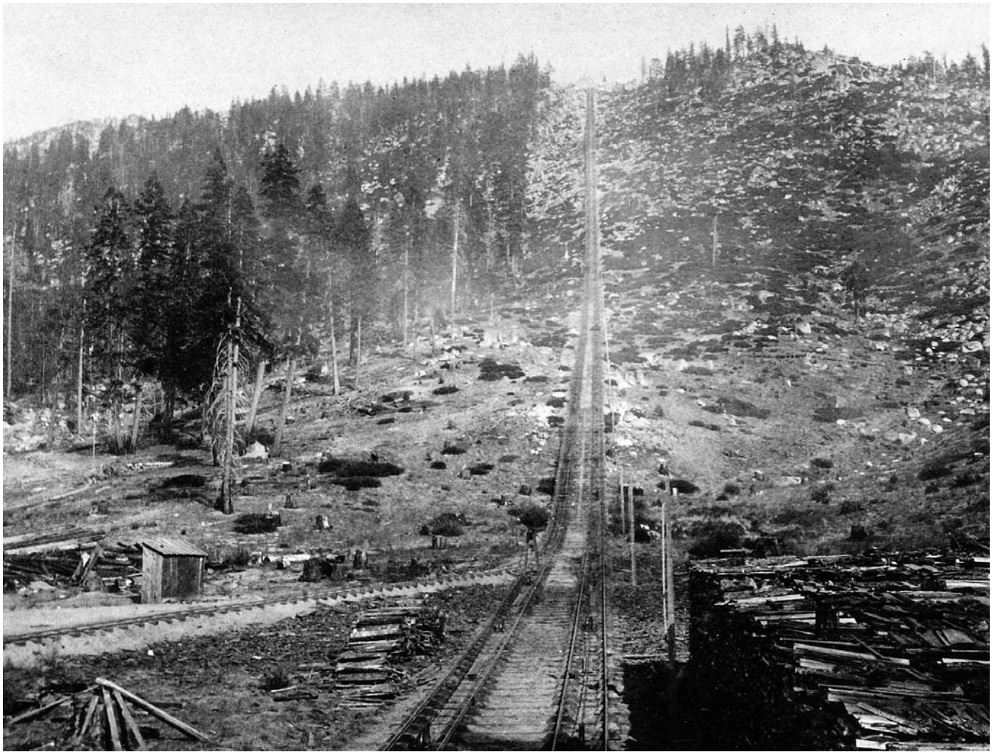
“The Great Incline of the Sierra Nevada,” around 1885. The incline rose 1,400 feet up the mountainside. From there, lumber was transferred to water flumes and transported to Lakeview just north of Carson City. It is now the location of Nevada Historical Marker #17.
