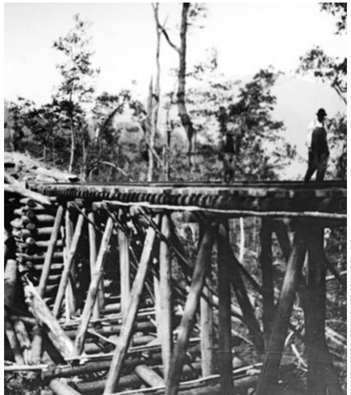
A trestle bridge on the logging railroad is about ready for use. In the excavations of the roadbed, we find lots of charcoal; sure evidence that the present generation of gigantic trees stands on the cinders of its mother trees.
