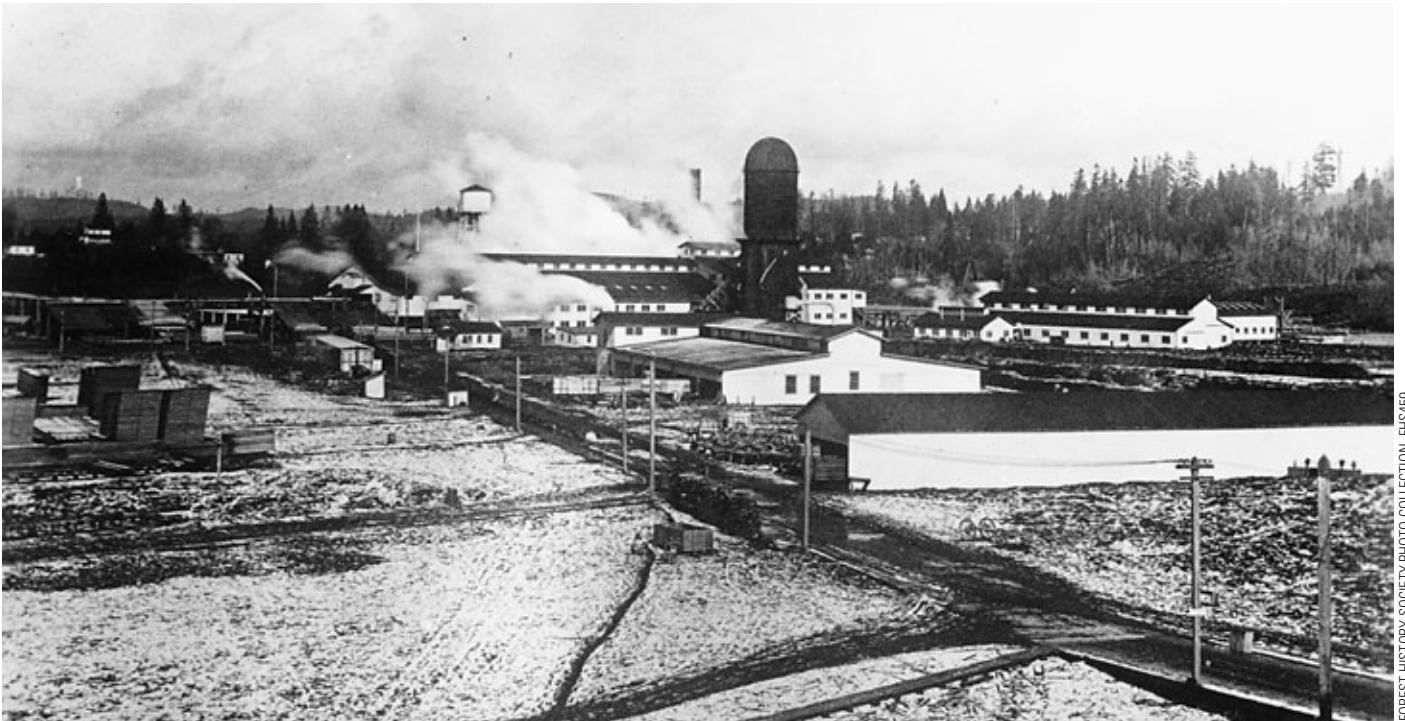
The C. A. Smith [Lumber Company's] sawmill at Marshfield (Coos Bay), Oregon, has a daily output of almost 1,000,000 feet b.m. of lumber. It is the largest sawmill in the U.S.A. There is but one difficulty: it is impossible to get rid of the offal of slabs, edgings, trimmings, and sawdust in its gigantic burning tower!
