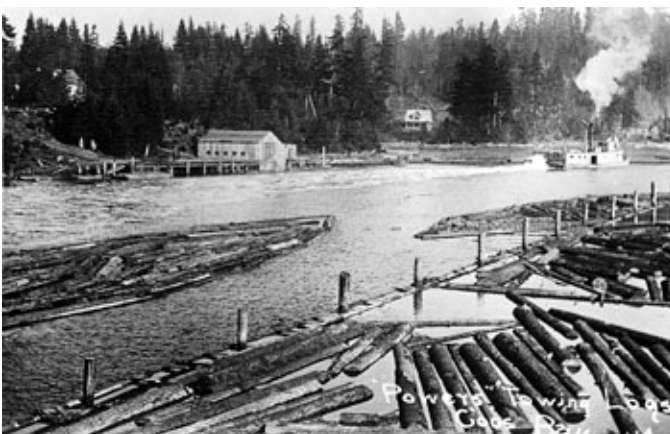
The logging train has been unloaded. The logs were dumped into the river and they are now towed, held together in a boom which looks like a triangular flat boat, to the sawmills of the C. A. Smith Lumber Company in Marshfield, Oregon.
