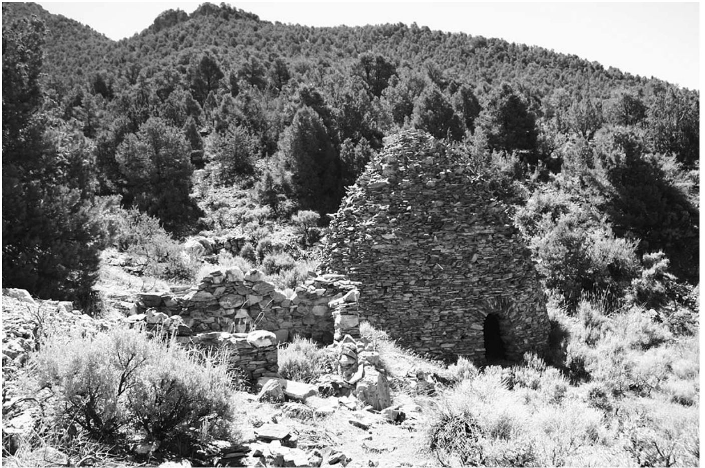
Like many of the kilns in Nevada, the Diamond City kilns are shaped like beehives.
