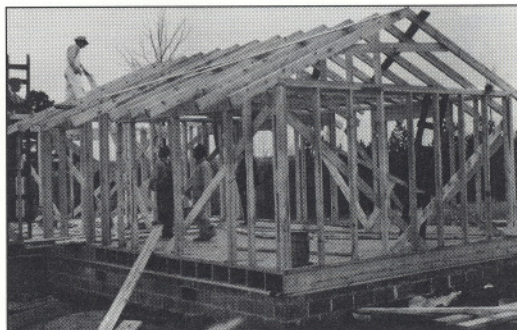
Typical construction using 2x4s. Photo from the Forest History Society archives.
