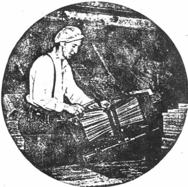
A packer builds up each bundle of shingles
