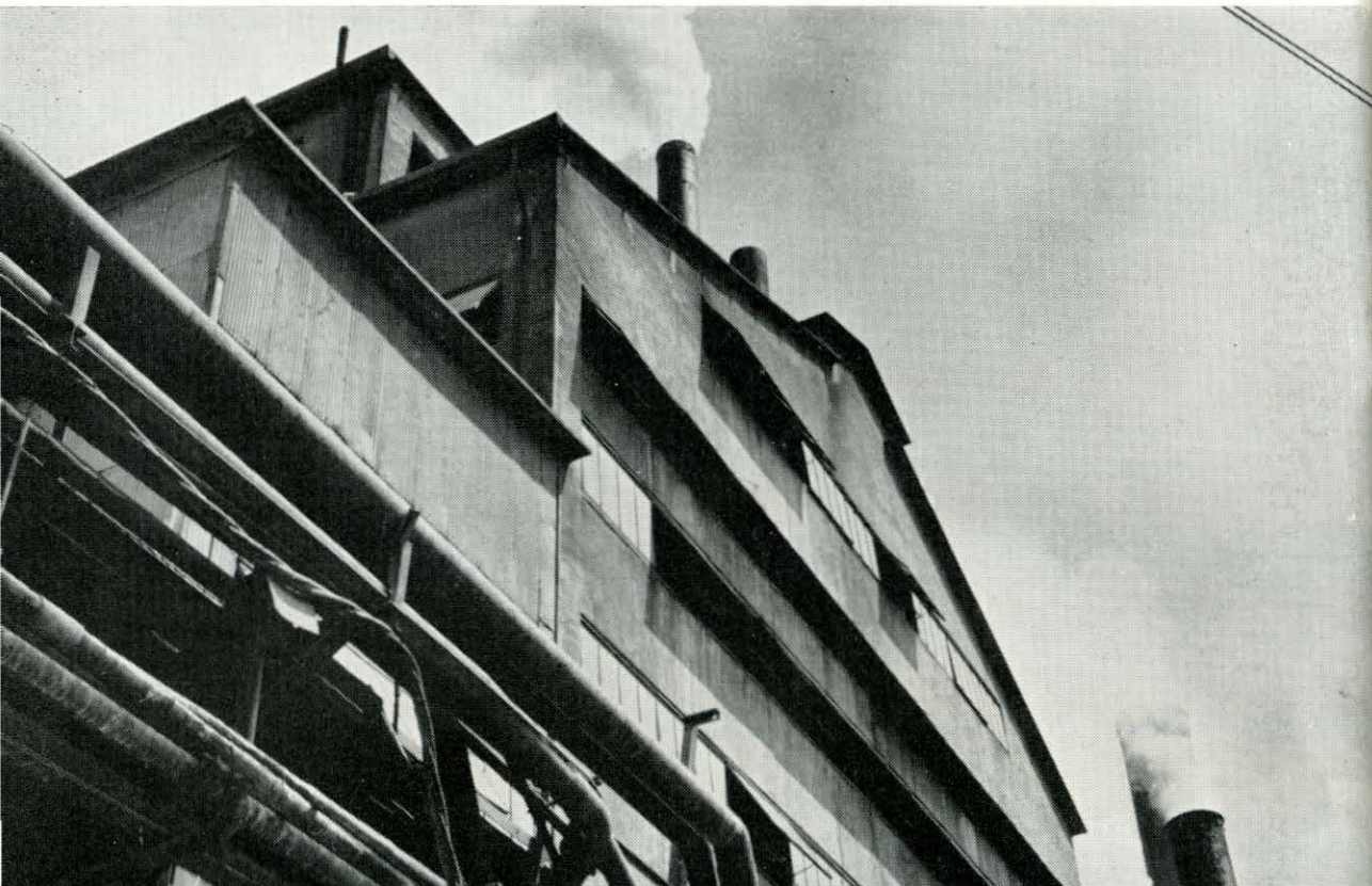
Smelter Furnace Building
