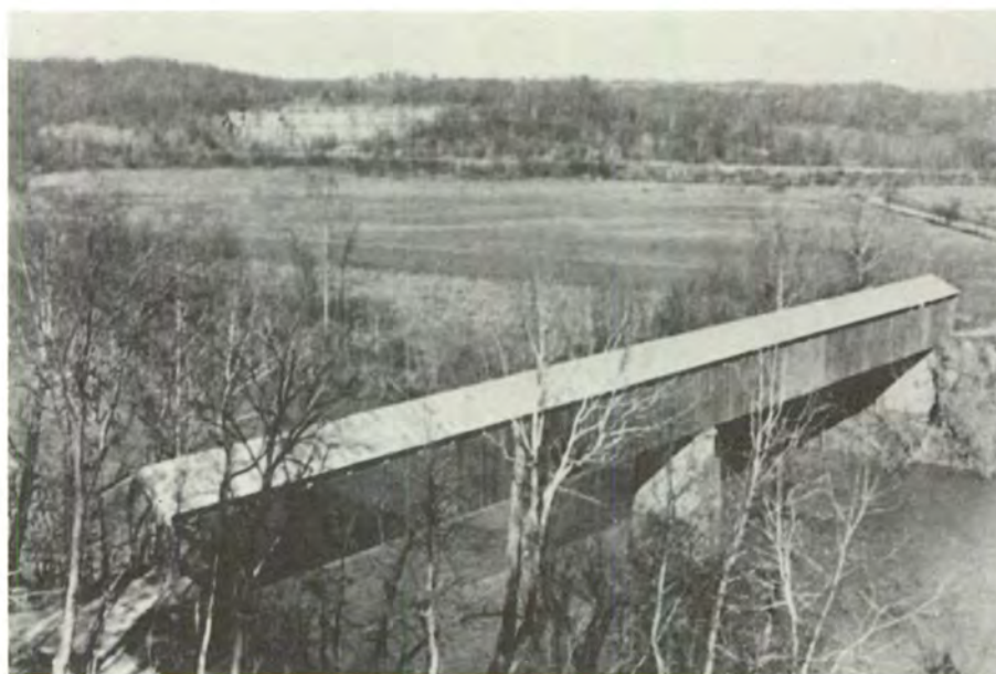
Figure 52: The 368 foot long covered bridge over the East Fork of the White River, Lawrence County, was built in 1884. Today it is listed on the National Register of Historic Places, and-- thanks to repairs and restoration--still used.
