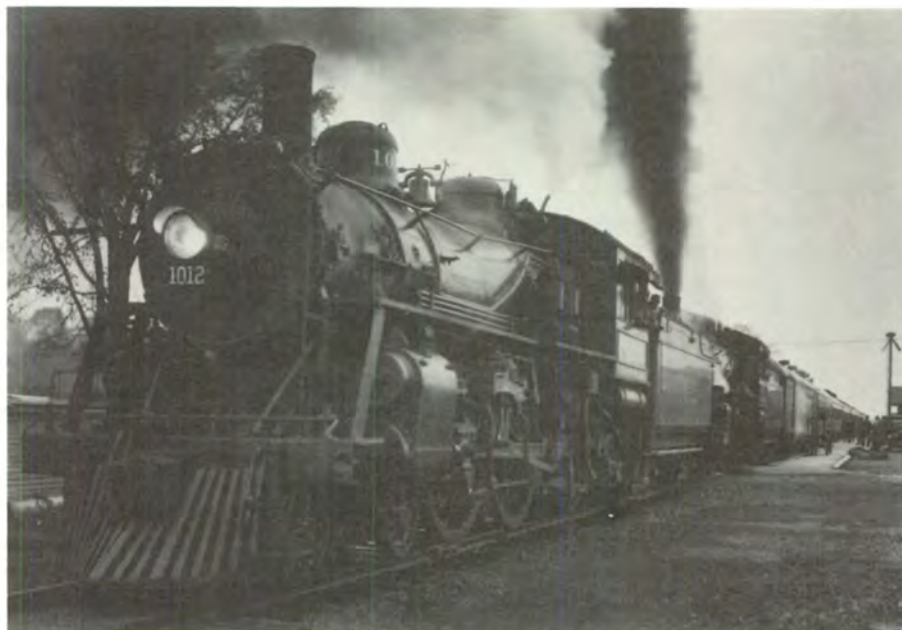
Figure 51: Double-header train at the Helmsburg depot in Brown County. The Illinois Central Railroad built a rail line across Brown County in 1905, opening up the county to quick access from the outside for the first time. The existence of this line helped encourage the development of the county's well-known artists' colony during the first part of the 1900s. Two large galleries and many artists are still present in Brown County.
