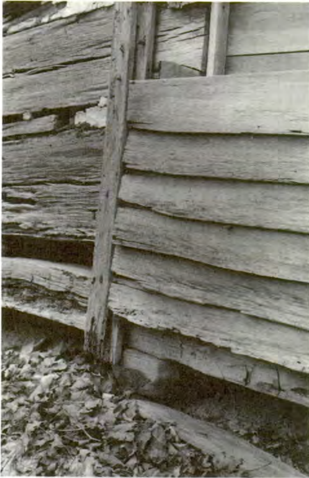
Figure 61: View of construction detail at the Waldrip House, showing the junction of the log room (left) and frame room (right), as seen from the south. Note the stone pier beneath the intersection of the two rooms.
