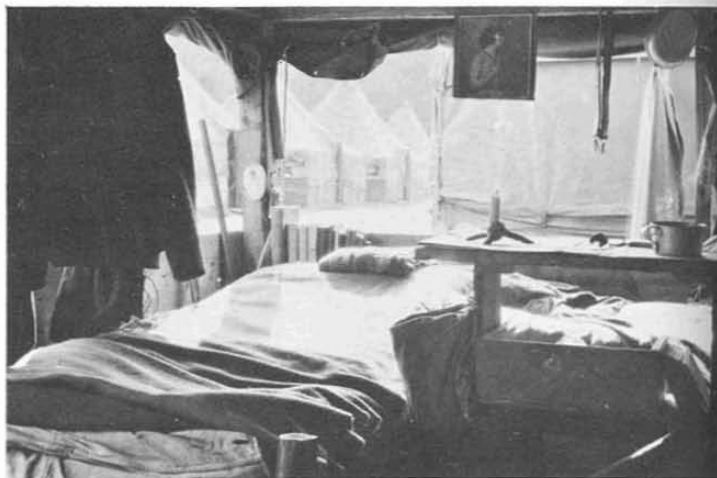
Log loading at Mortumier, 1918. Above: Kephart's bunk at Mortumier Camp, 1918.
