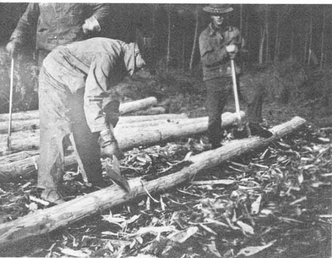
Pole operations at Mortumier, 1917.
