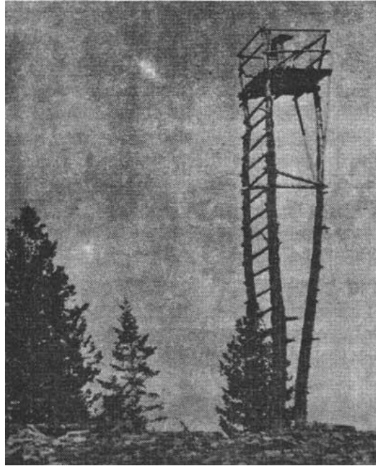
Old Gold Peak Tower on day it was condemned — August 22, 1920. This tower originally was built by one man without assistance. Missoula (now Lolo) N. F.
