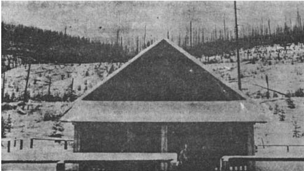
Sylvanite Ranger Station a few years after the 1910 fire, Kootenai National Forest. J.K. John Brobst in picture.
