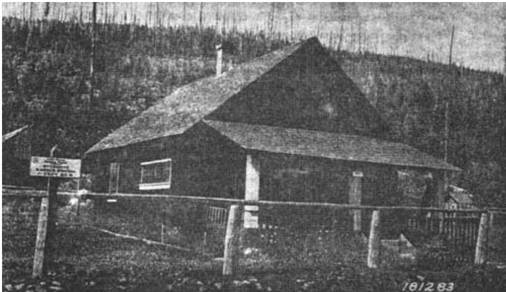
Sylvanite Ranger Station, Kootenai National Forest, August 1923. Area behind building was burned over during 1910 fire.
