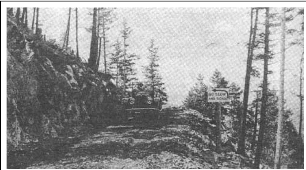
LIBBY - TROY ROAD in Montana, Kootenai National Forest, 1915. Typical rock excavation on improvement.
