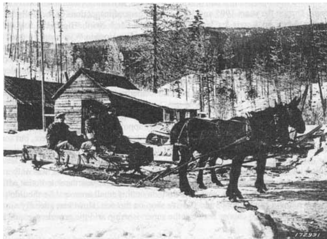
Government team and scaler's cabin at Beardmore's Tunnel Camp, Kaniksu National Forest. Howard Drake and Hank Ogsden in seat. 1923.
