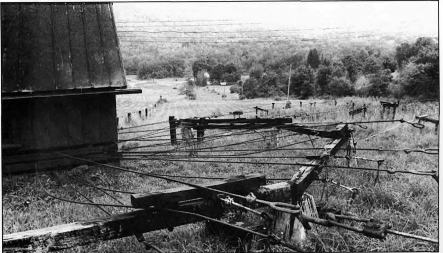
Cline Oil Co. central power, still operating at Degolia, Pa., 1994. Phil Ross
