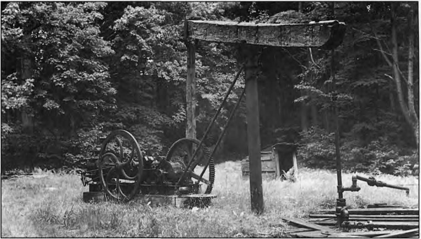
The Forest Service began purchasing much of the surface area of the Middle Field in 1923. The early Allegheny National Forest hosted a well-established producing industry. Pictured here is a Barcroft" or "Blaisdell" compressed-air pumping rig, in 1926. Note the modified Farrar & Trefts steam engine. USDA Forest Service
