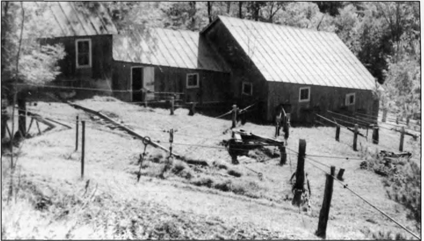
Late design South Penn central power, Bradford Field, 1970. Mike Fuoco
