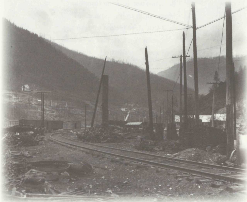
1910 Coeur d'Alene NF. Burned over area in Wallace near the ruins of the foundry. The cottage on the hillside (left) is the only one left standing in town. Photo by R.H. McKay.
